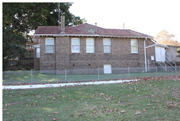
Figure 3 South elevation of Wansey Cottage featuring distinctive Federation style detailing including brickwork, terracotta tiled roof, timber joinery and exposed rafters. (Source: GML 2015)
