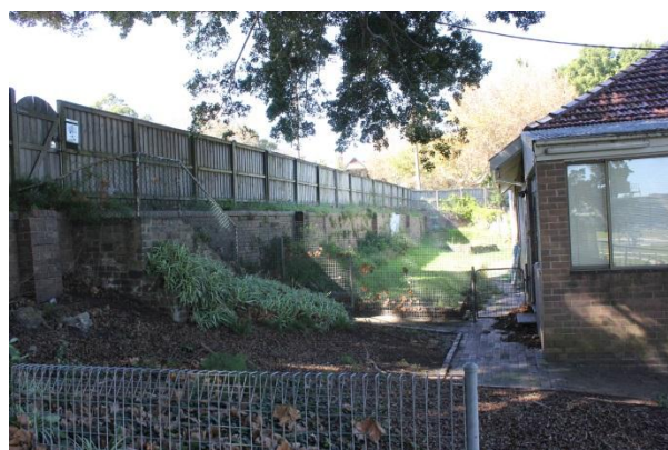
Figure 5 View along the northern side of Wansey Cottage and the access stairs to Alison Road. (Source: GML 2015)
