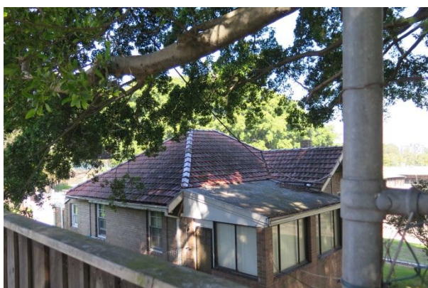
Figure 4 View of Wansey Cottage from Alison Road showing the c1960s verandah addition. (Source: GML 2015)
