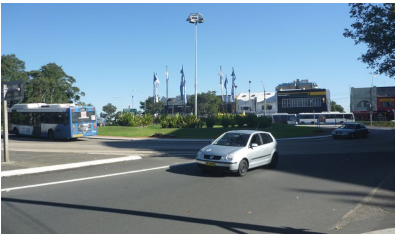
Figure 16.15 View of the existing Nine Ways intersection
