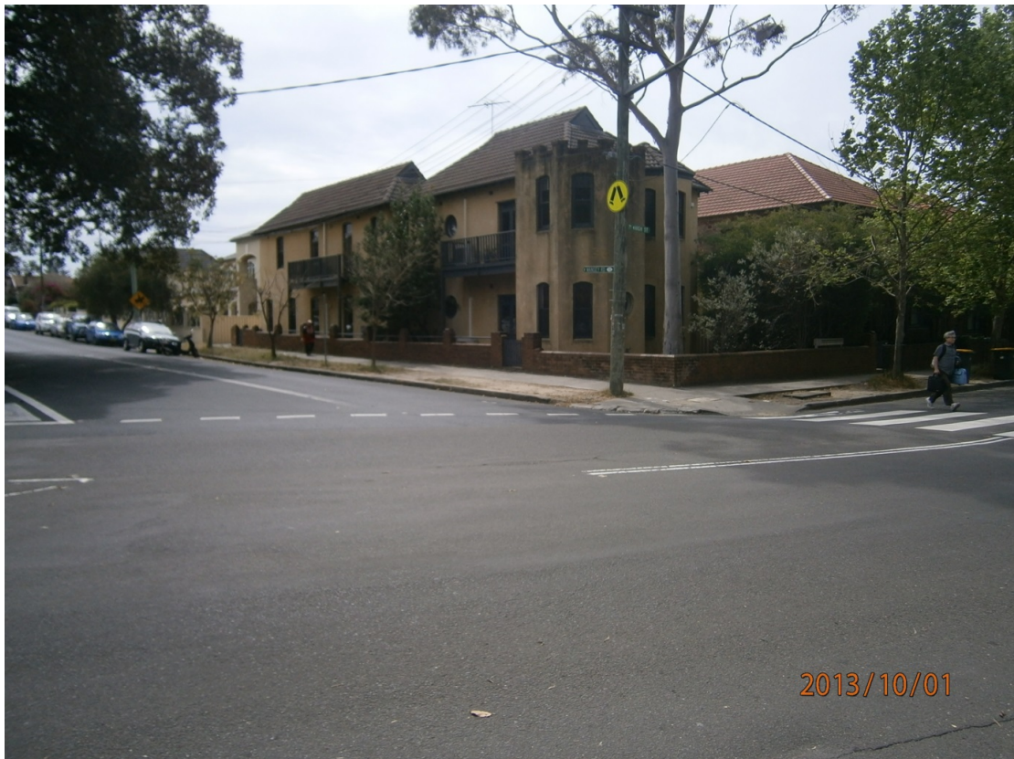
Photo P2 – High Street/Wansey Road intersection, view north from west side of intersection
