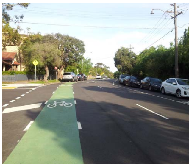
Figure 4 Example of On-Road Cycleway with Green Paint
