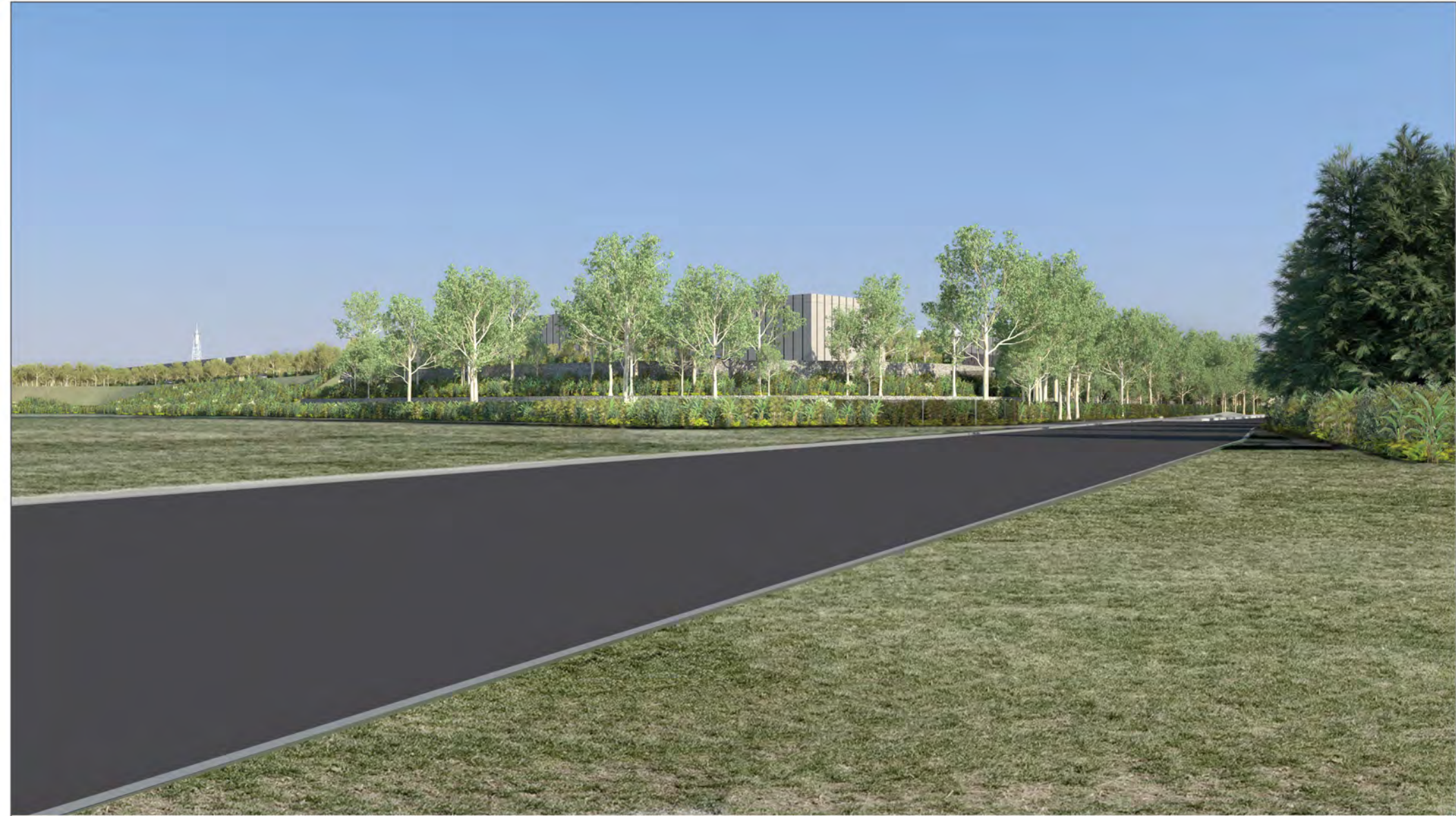
CAMERA 6 – Eye level view from north west (future Hambledon Road north)
