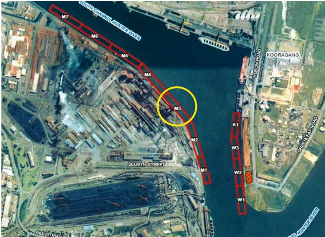
FIGURE 2 LOCATION OF THE BERTH EXPANSION WORKS, AS INDICATED BY THE YELLOW CIRCLE
