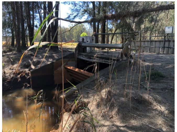
Photograph 8 Hydraulic creek flow gate located north of the proposed WWTP (Segment 1)
