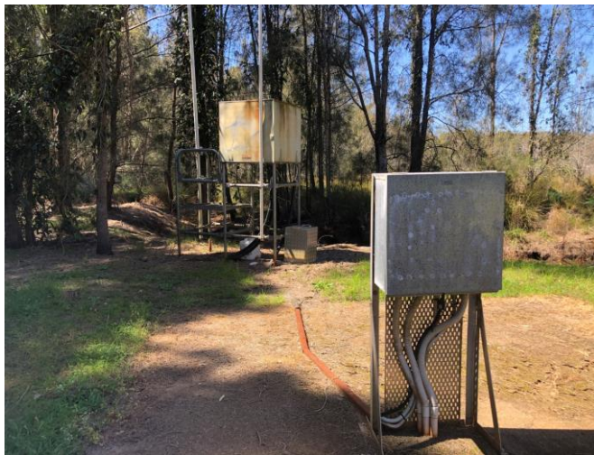
Photograph 7 The control box and hydraulic oil hopper for the hydraulic creek flow gate use for ASS management located north of the proposed WWTP (Segment 1)
