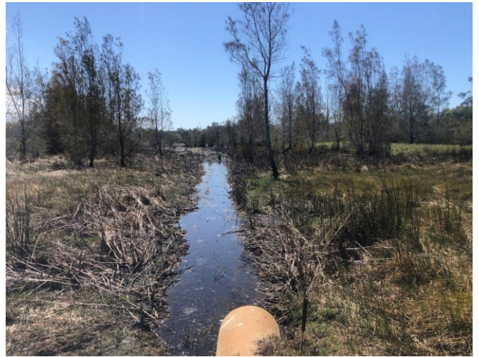
Photograph 6 Swale for inflow to the wetland (Segment 1)
