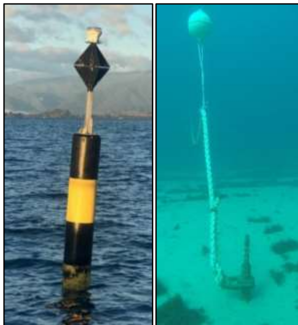
Figure 6: South Coast Mariculture cardinal navigation marker above and below surface (Source South Coast Mariculture 2019)
