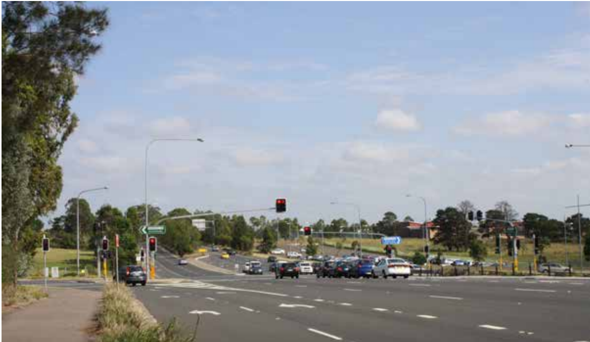
Figure 23 – View 1 - Along Windsor Road (looking north)
