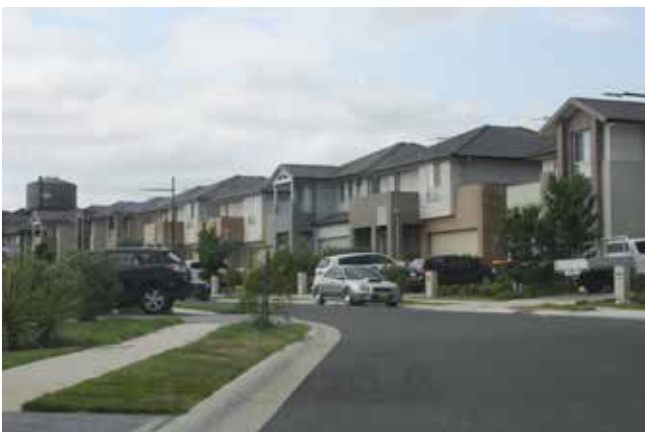
Figure 5 – Typical built form in the area around the proposed bridge
