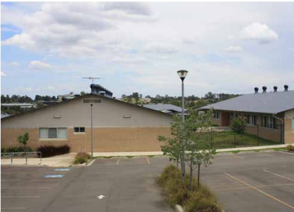
Figure 35 –View 7- from Withers Road (looking west). The view is across Rouse Hill High School Source: Studio GL
