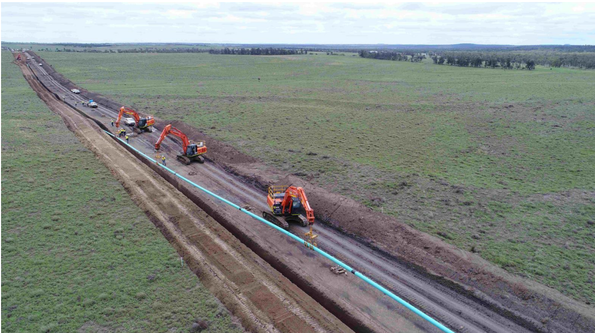
Figure 3.12 Example of lowering in the pipeline using side boom tractors
