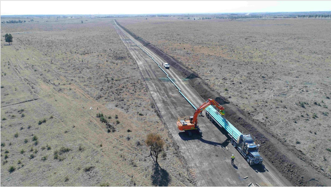
Figure 3.10 Example of pipeline stringing
