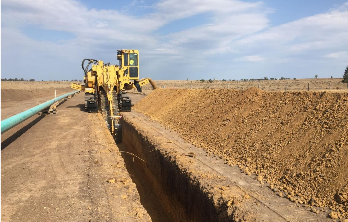
Figure 3.11 Example of trenching and spoil placement
