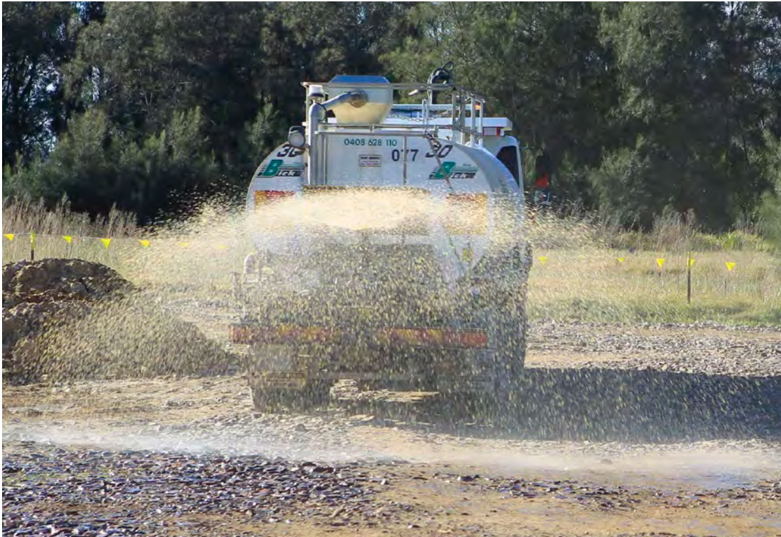
Photo courtesy of Roads and Maritime Services.
