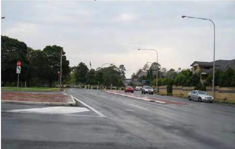
Photo 4.4 Old Northern Road, looking north from intersection with Terminus Street
