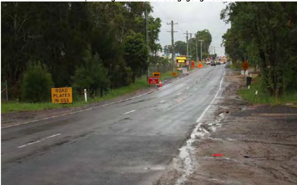
Photo 4.12 Schofields Road, looking west toward Cudgegong Road
