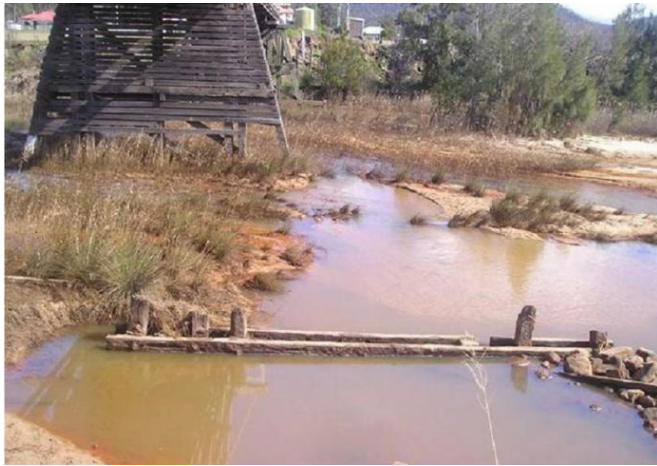
Non-Aboriginal heritage: Remnant bridge piers
