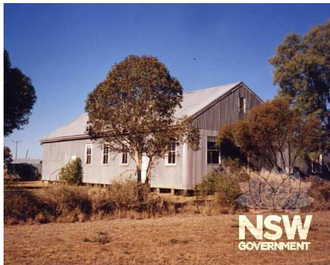
Non-Aboriginal heritage: shearing shed
