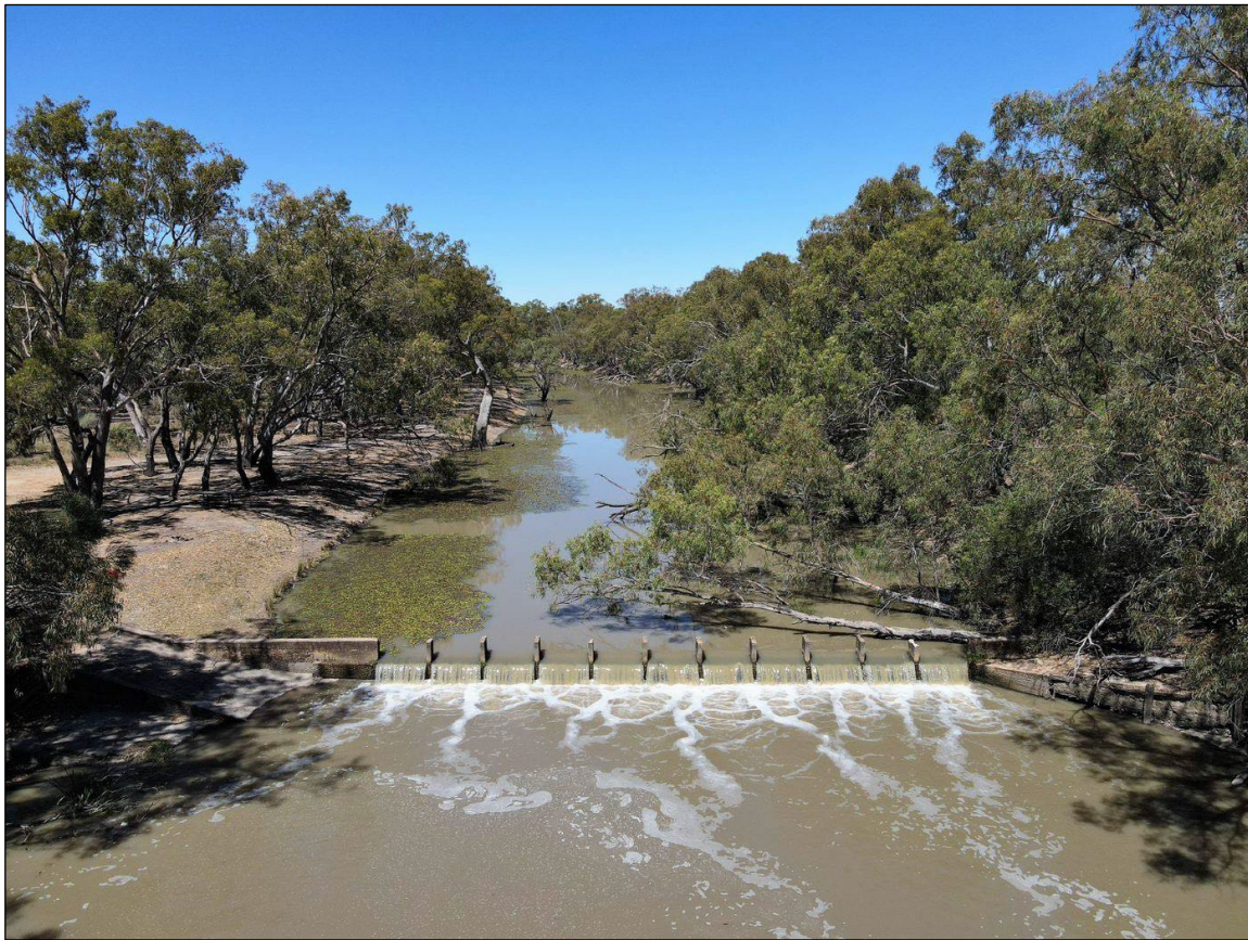
Figure 6 | Existing Wanganella Weir (Source: EIS)
