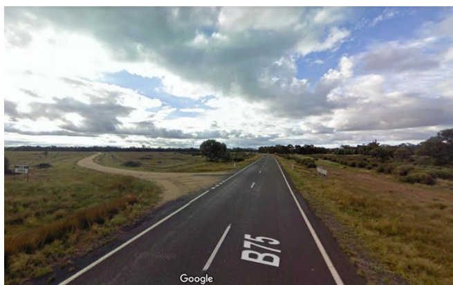
Figure 15.1 Cobb Highway View facing north, approaching intersection with Zara Road near Wanganella
