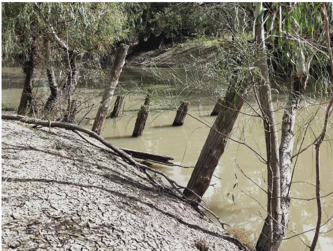
Figure 13.5 Timber uprights and posts on the east bank, facing southwest
