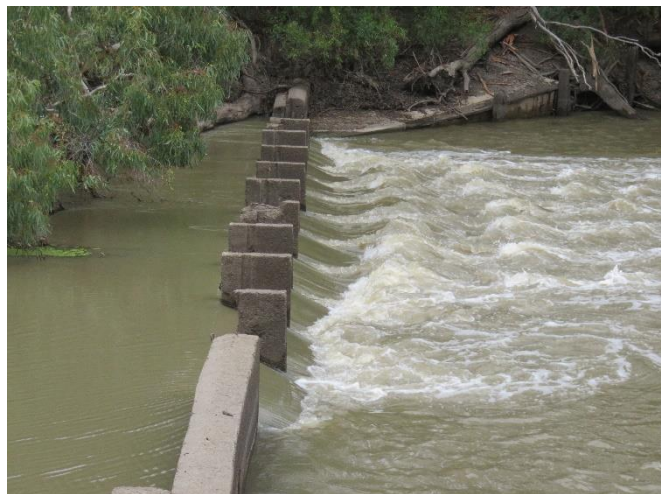
Figure 2.2 Examples of deterioration and missing drop boards at the existing Wanganella Weir
