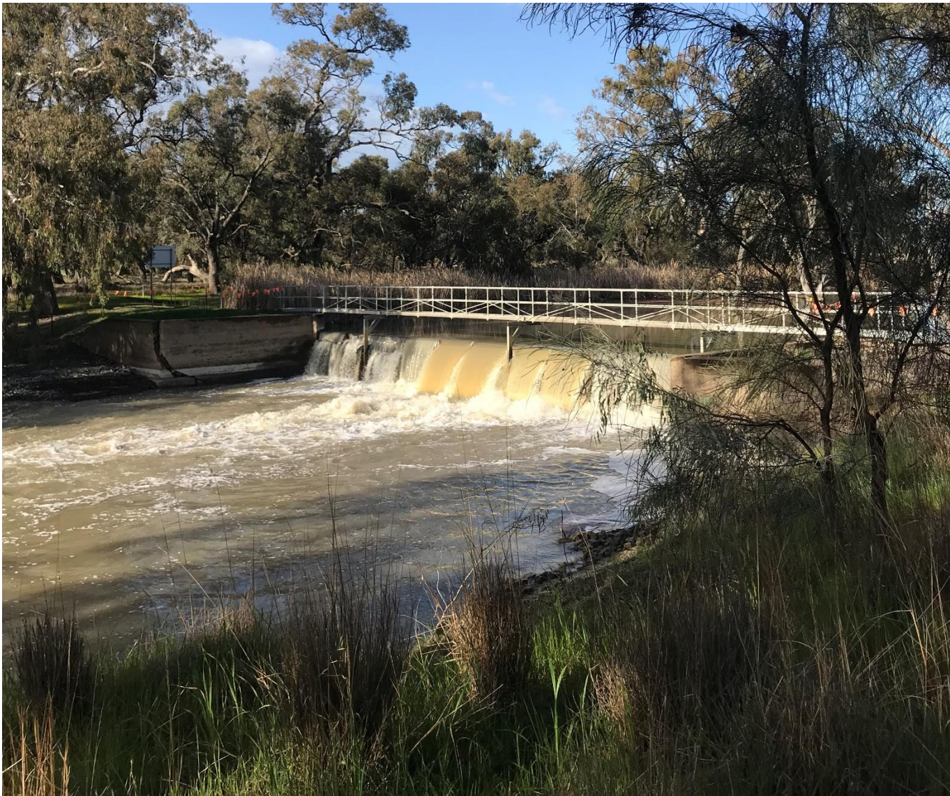
Figure 17.23 VP5: Hartwood Weir looking south– existing view
