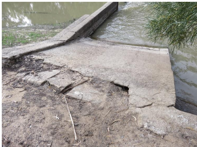
Figure 2.2 Examples of deterioration and missing drop boards at the existing Wanganella Weir
