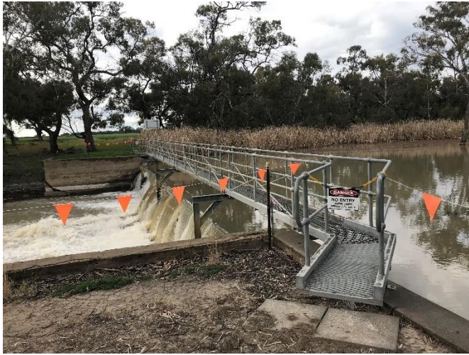
Figure 17.13 Hartwood Weir footbridge and signage
