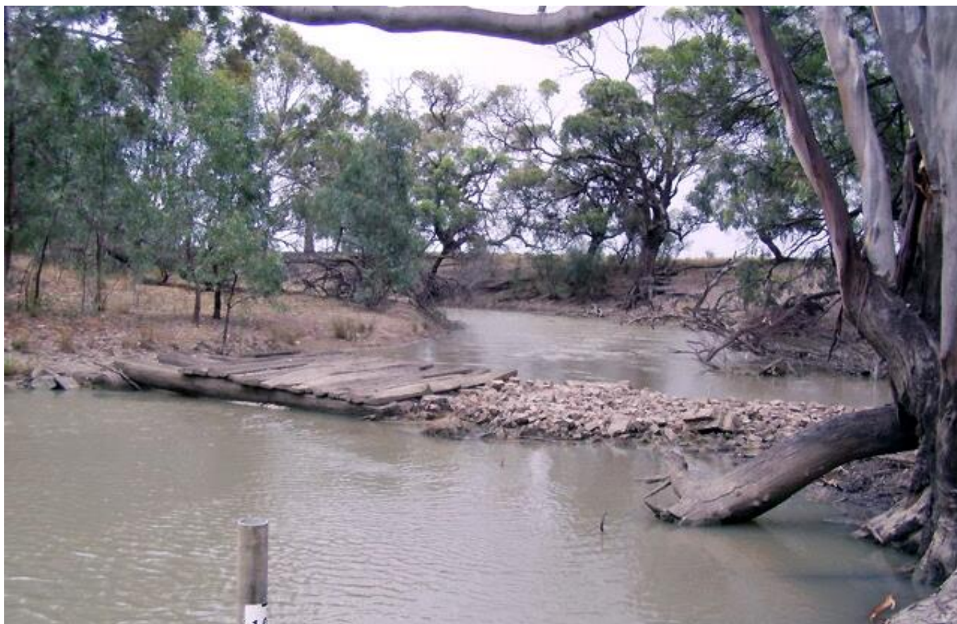
Figure 13.4 DCCEEW photograph of the Old Bridge and stone crossing during a dry period, near Hartwood Weir
