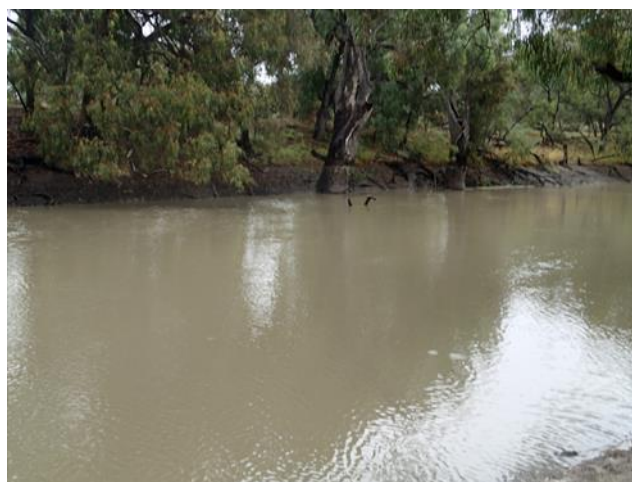
Figure 9.8 100 metres downstream of Wanganella Weir showing stable channel banks, and clear high water mark
