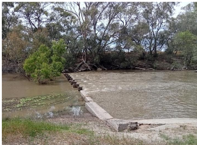
Figure 9.5 Looking across channel at Wanganella Weir from right hand bank
