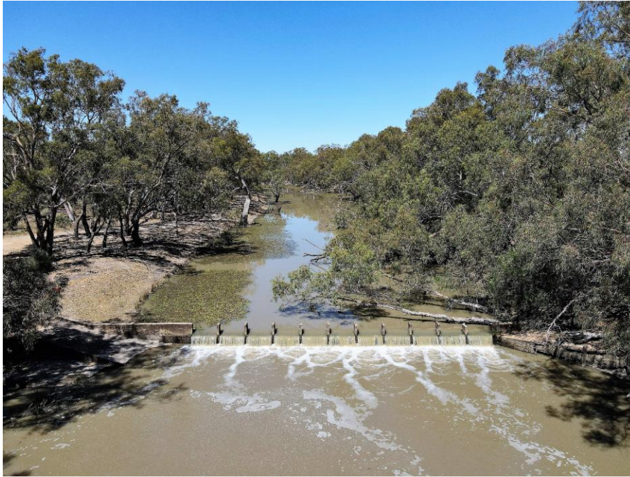
Billabong Creek @ Wanganella Weir
