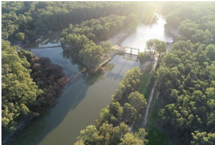
Murrumbidgee River @ Yanco Fixed Crest Weir (left) and Yanco Weir (right)
