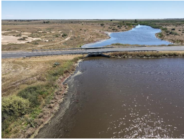
8 Mile Creek Southern Regulator
