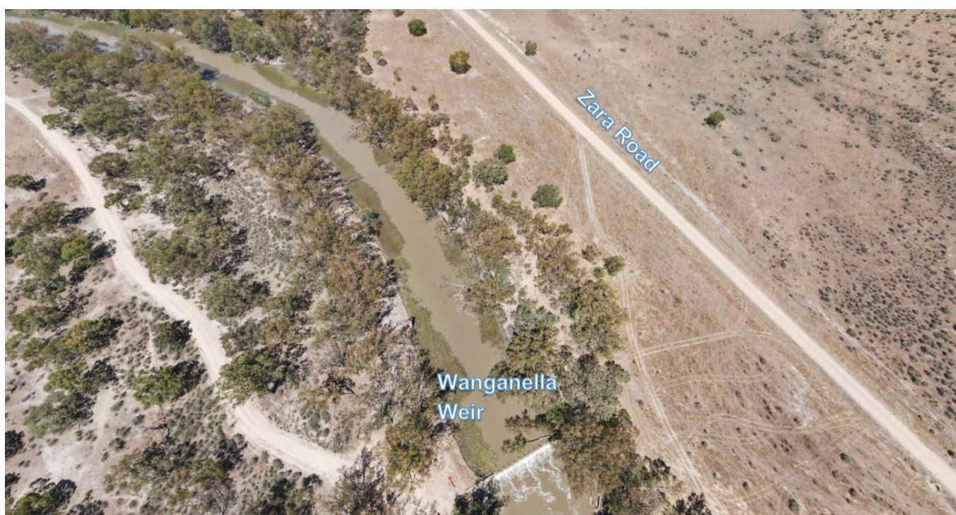
Figure 3.6 Zara Road, view facing south east from Wanganella Weir
