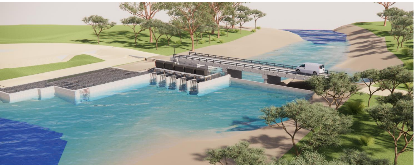
Figure 1.2 Indicative layout of a regulator
