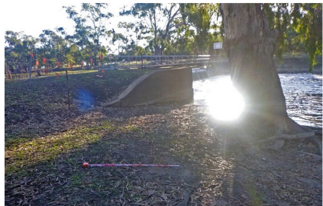
Figure 4-4. View of Hartwood Weir, facing northwest (Photograph by Brendan Wong)
