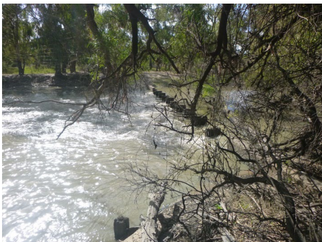
Figure 4-26. View of Wanganella Weir from the south bank, facing northeast (Photograph by Brendan Wong)
