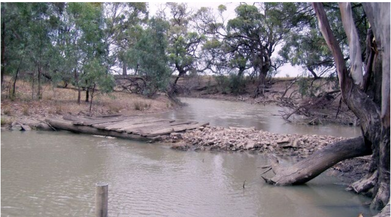
Figure 4-12. NSW DCCEEW photograph of the Old Bridge and stone crossing during a dry period
