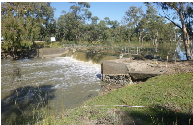
Figure 4-3. View of Hartwood Weir, facing southeast (Photograph by Brendan Wong)
