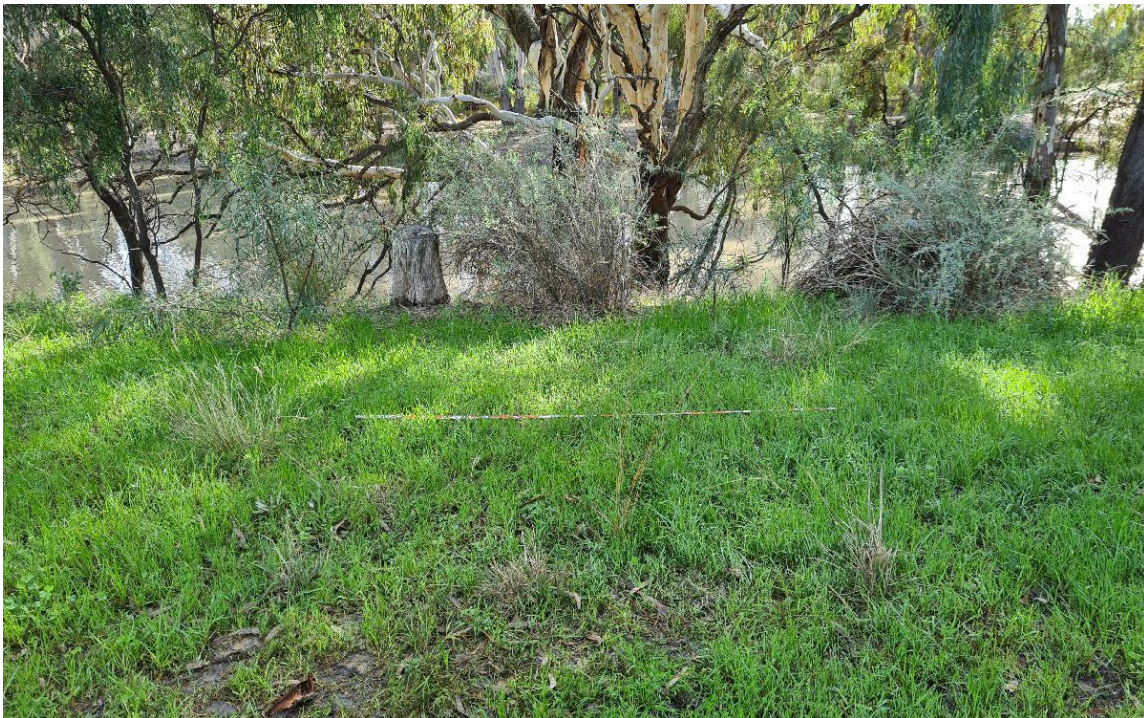
Figure 7.49 North-facing view of the proposed Wanganella Weir construction zone. Photograph taken on 13 July 2023 by Madelaine Firth.
