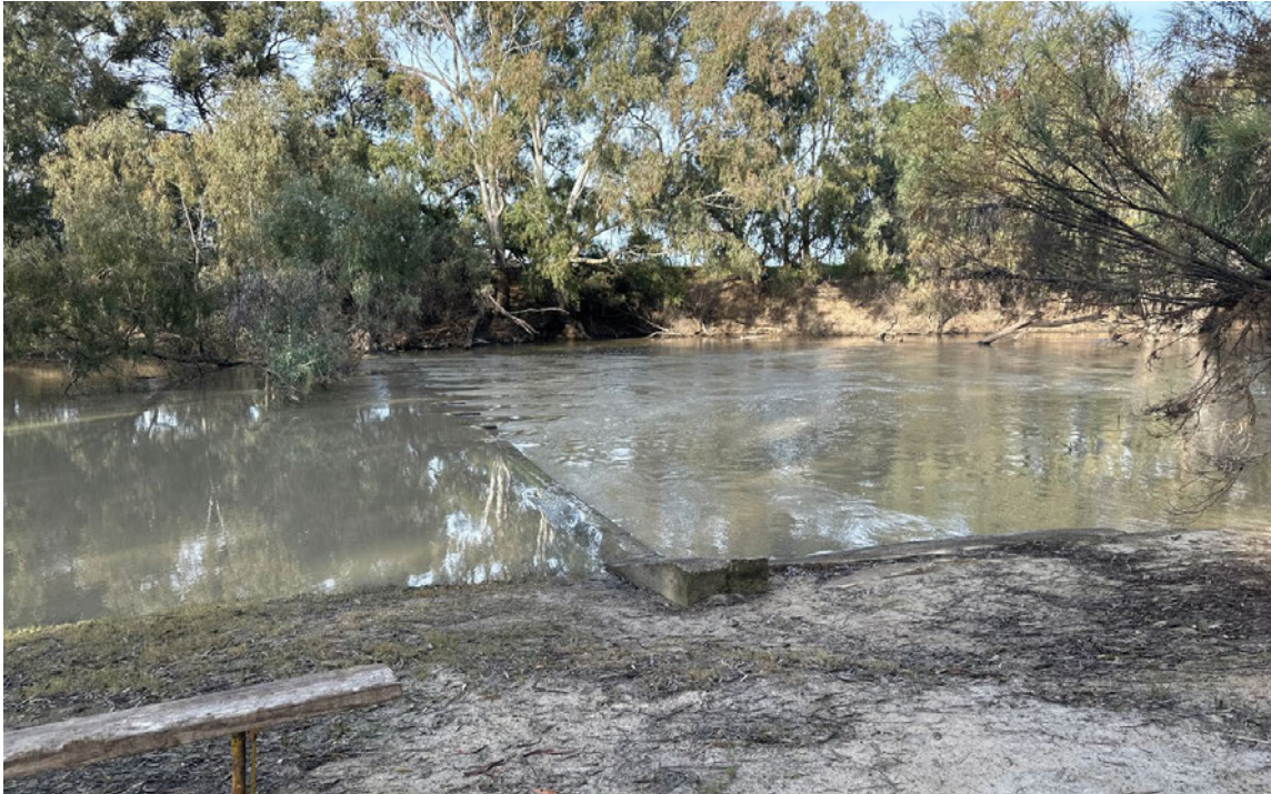
Figure 7.47 South-facing view of existing Wanganella Weir and construction zone. Photograph taken on 13 July 2023 by Madelaine Firth.
