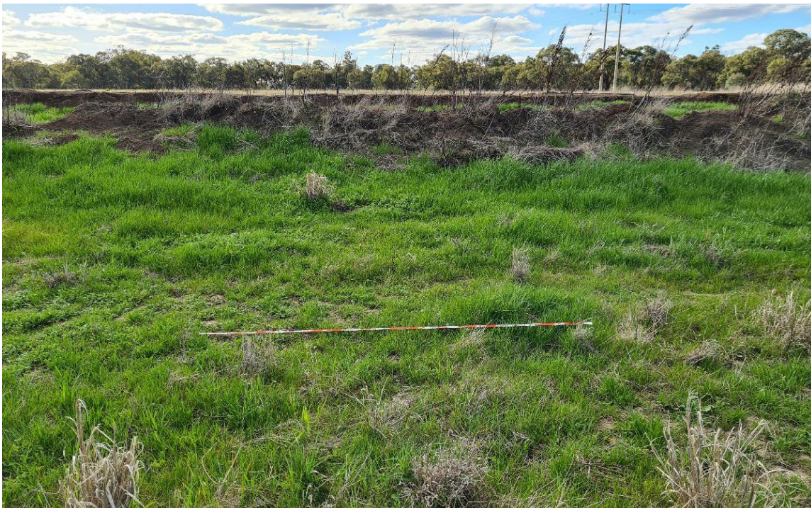
Figure 7.3 North-facing view of channel and levy construction disturbance near Hartwood Weir. Photograph taken on 13 July 2023 by Nicole Monk.
