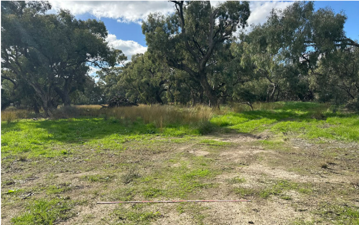
Figure 7.19 North-east-facing view of access track within Hartwood Weir construction zone. Photograph taken 13 July 2023 by Nicole Monk.
