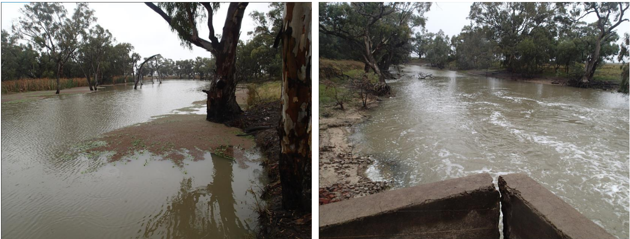
Looking at channel upstream of existing weir. Stable channel banks with reeds at margins.
