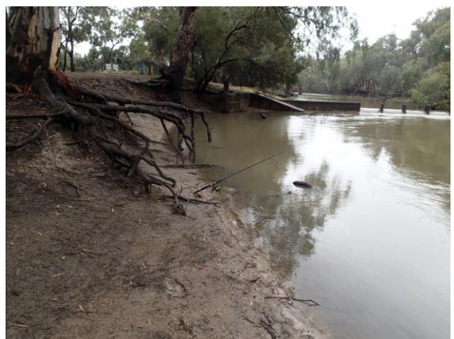
Looking upstream at bank erosion that has occurred immediately downstream of Wanganella Weir.
