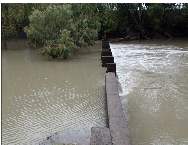
Looking across channel at Wanganella Weir from right hand bank.
