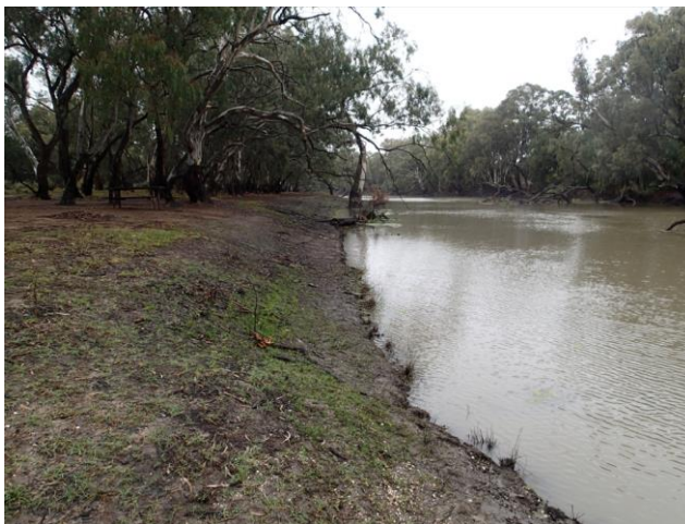
Looking at channel upstream of Wanganella Weir. Minor erosion/notching of banks in weir pool.
