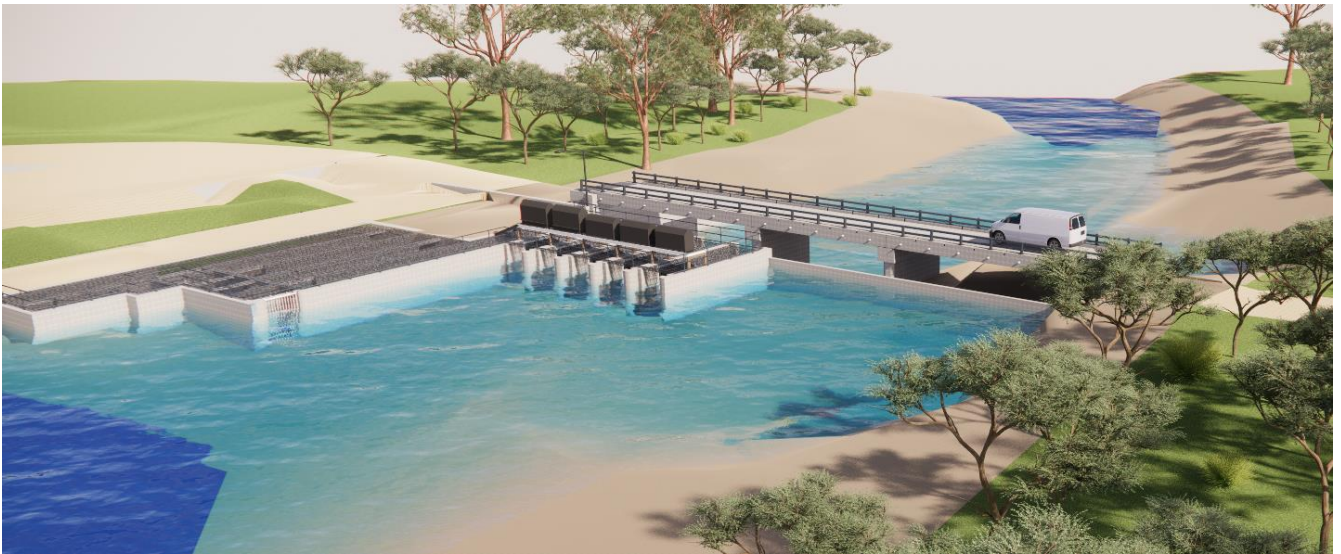
Figure 1-2 Indicative layout of a regulator
