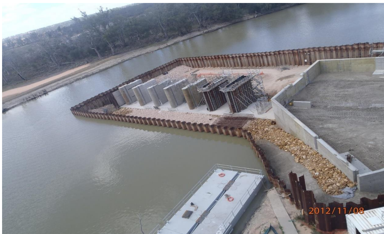
Figure 4-2 Example of a temporary partial cofferdam configuration.
