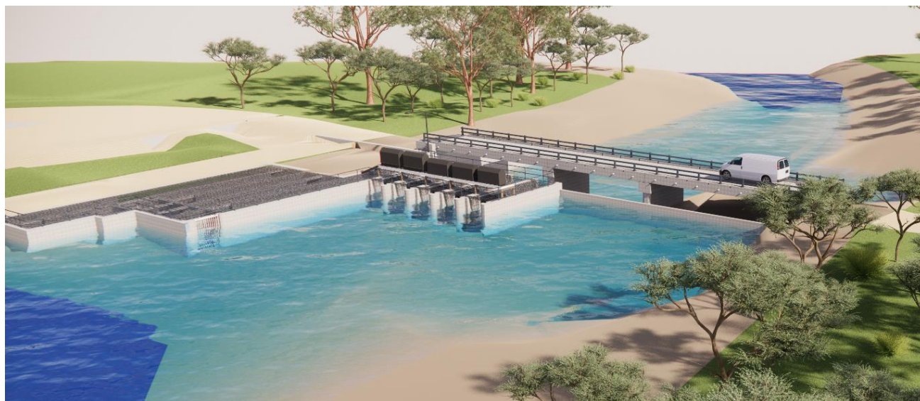
Figure 1-4 Indicative layout of a regulator.
