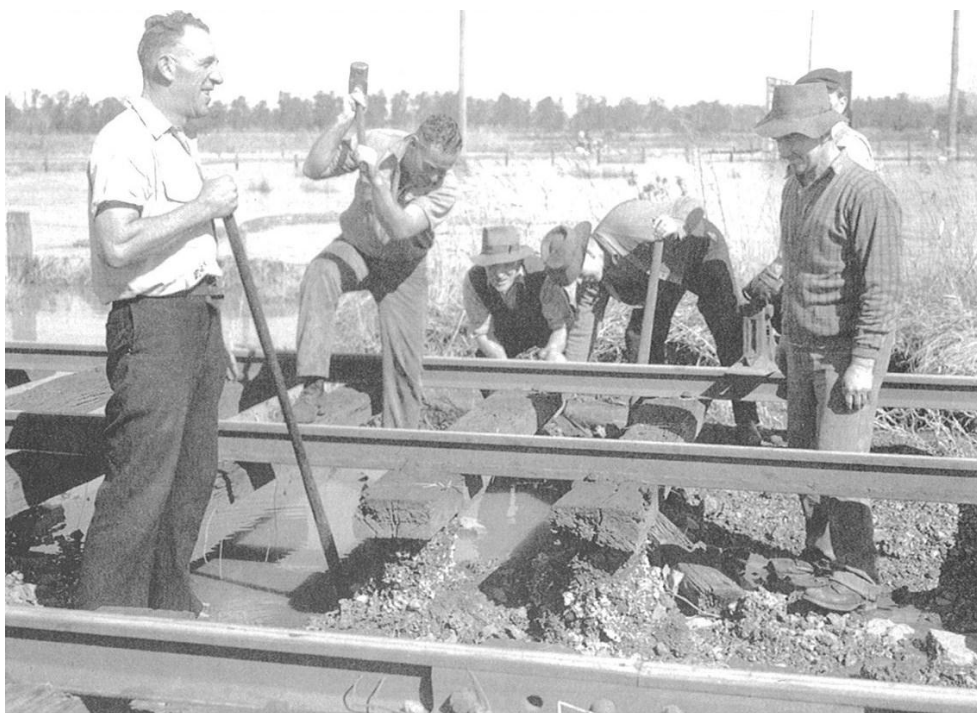
Figure A.2 Railway fettlers repairing the railway line near the Hexham signal box on 11 August 1952 (Source: Newcastle Region Library, in McKillop and Sheedy 2008:136).
