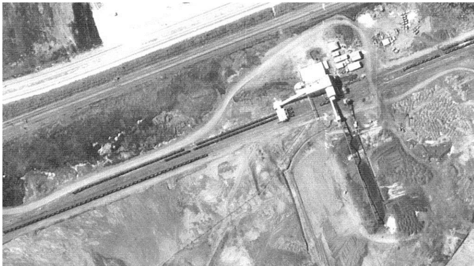
Figure A.27 Detail of the 1965 aerial photograph showing J&A Brown Hexham Coal Washing Plant.
