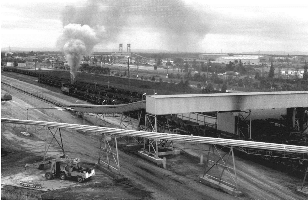
Figure A.28 The stacking out and reclaim coal conveyors. The lower, 'thin' conveyor is the stacking out coal conveyor, while the larger, upper conveyor is the incoming reclaimed coal conveyor. Note the concrete foundations for the conveyor stanchions (Source: Lockett 2004:371).
