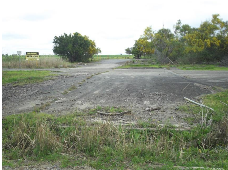
Photograph 3: Area of former buildings, likely associated with the Hexham Coal Preparation Plant
