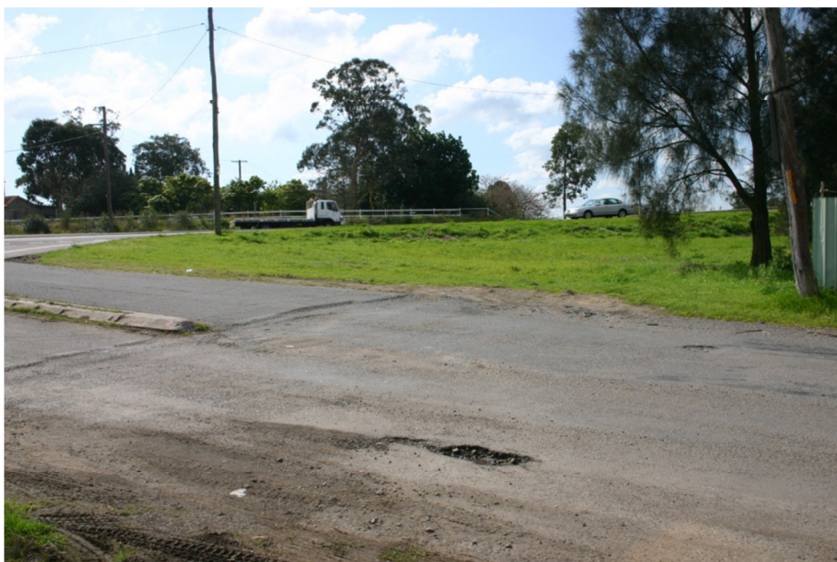
Figure 6.10 Rise of land on northern side of Woodlands Close intersection with New England Highway.
