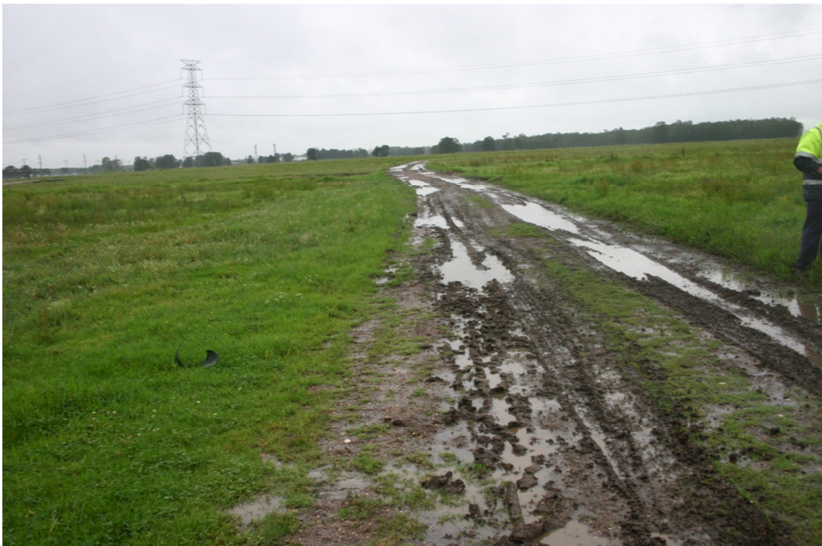
Figure 6.12 Area of exposure created by vehicles to access pipeline area.
