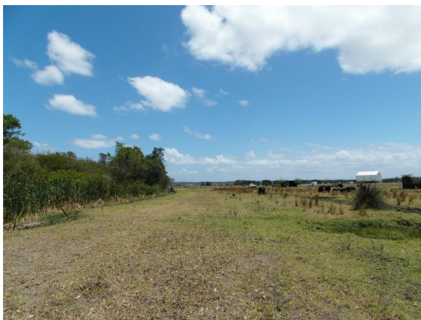
Figure 2.1 View west along the railway corridor with vegetation, drainage channel and embankment to the left.
