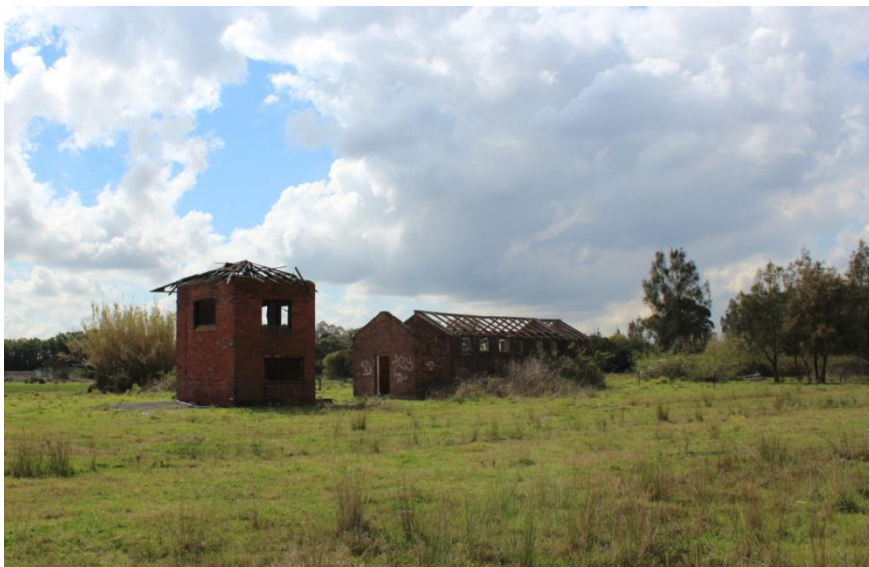
Figure 2.12 Two brick structures east of the corrugated steel structures and adjacent to the SEPP 14 lands.
