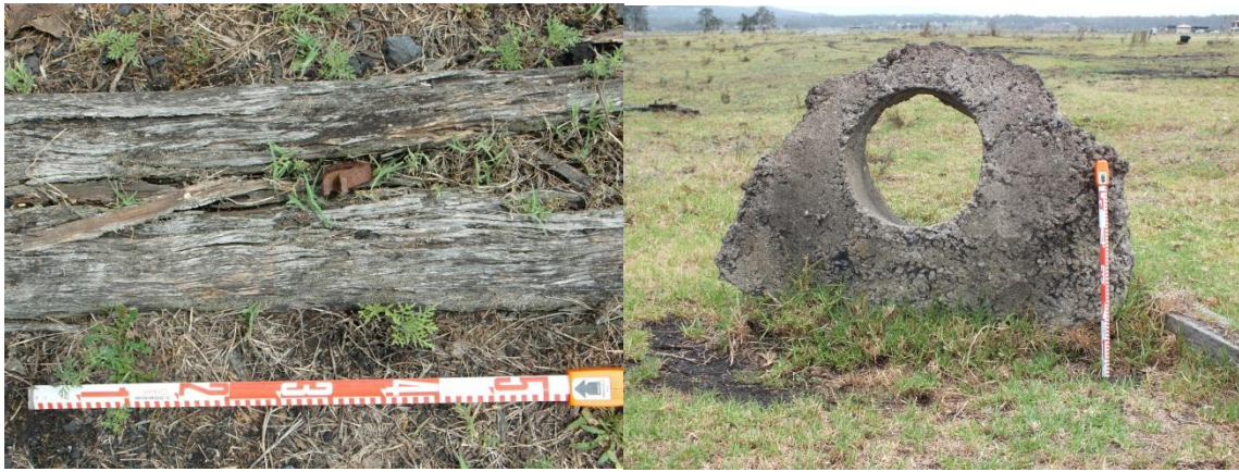
Figure 2.7 Detail of split pin in a sleeper and the concrete base within the rail corridor.
