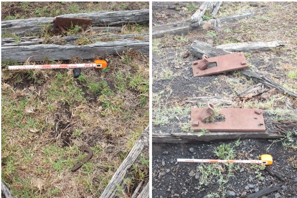
Figure 2.6 Detail view of sleepers base plates and split pins.
