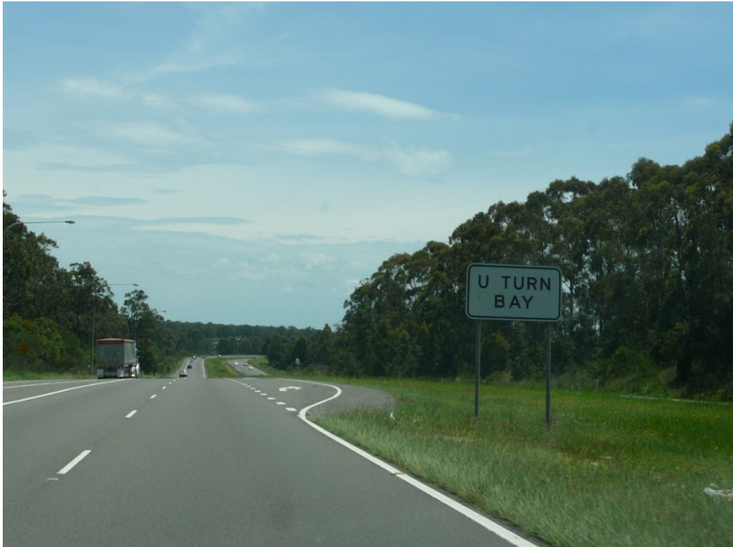
Figure 2.17 New England Highway, looking northbound towards U-turn bay
