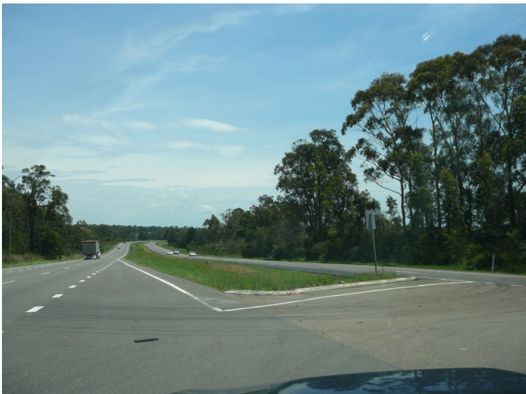
Figure 2.18 New England Highway U-turn bay, looking northbound towards Maitland
