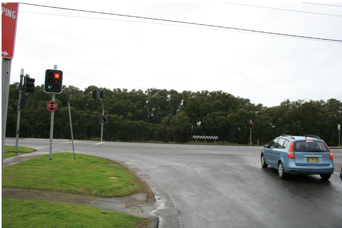
Figure 2.8 Maitland Road (Pacific Highway)/Shamrock Street intersection, looking east looking toward Maitland Road
