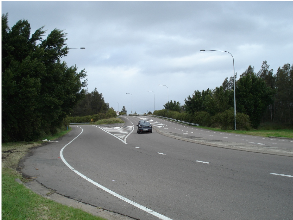
Figure 2.12 Tarro Interchange, looking south from Anderson Drive
