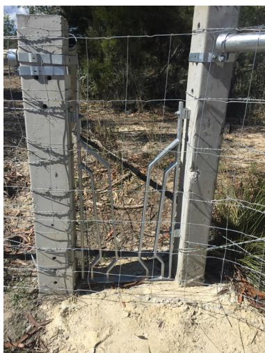
Plate 9. Emu gate blocked using mesh fencing wire to keep in sheep or goats.
