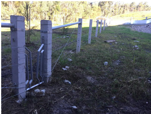
Plate 5. Completed hybrid fence and emu gate Section 3 Chaffin Creek (chainage 52423)
