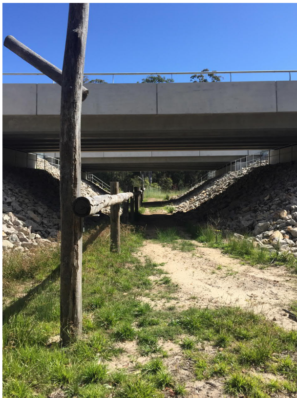
Plates 7 and 8. Completed crossing zones at end of construction showing fauna furniture and exclusion fencing to prevent emus entering the road corridor and direct to crossing zones
