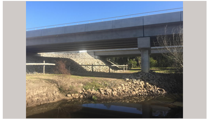
Plate 6. Completed Emu crossing zone Pillar Valley Creek floodplain Section 3 (chainage 47841)
