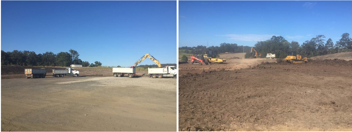
Figure 21 Hardstand removal, McIntyres Lane ancillary facility
