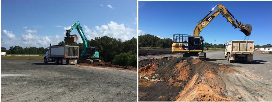
Figure 28 Broadwater hardstand removal
