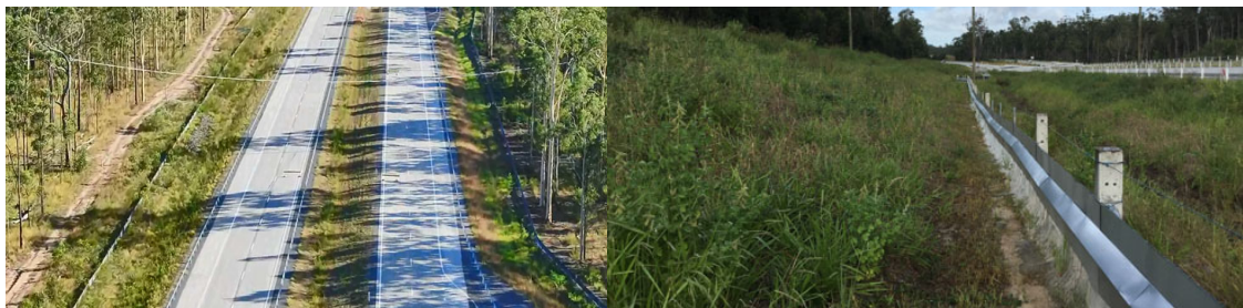
Figure 36 Fauna rope bridge and permanent fauna fencing examples, Section 7
