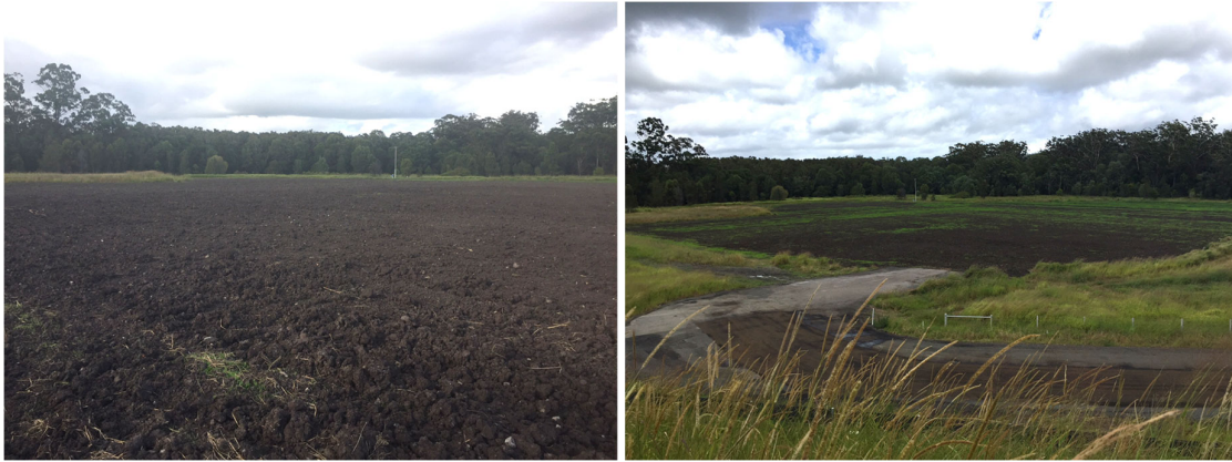
Figure 26 Iluka Road topsoil and seeding completed / partial grass strike
