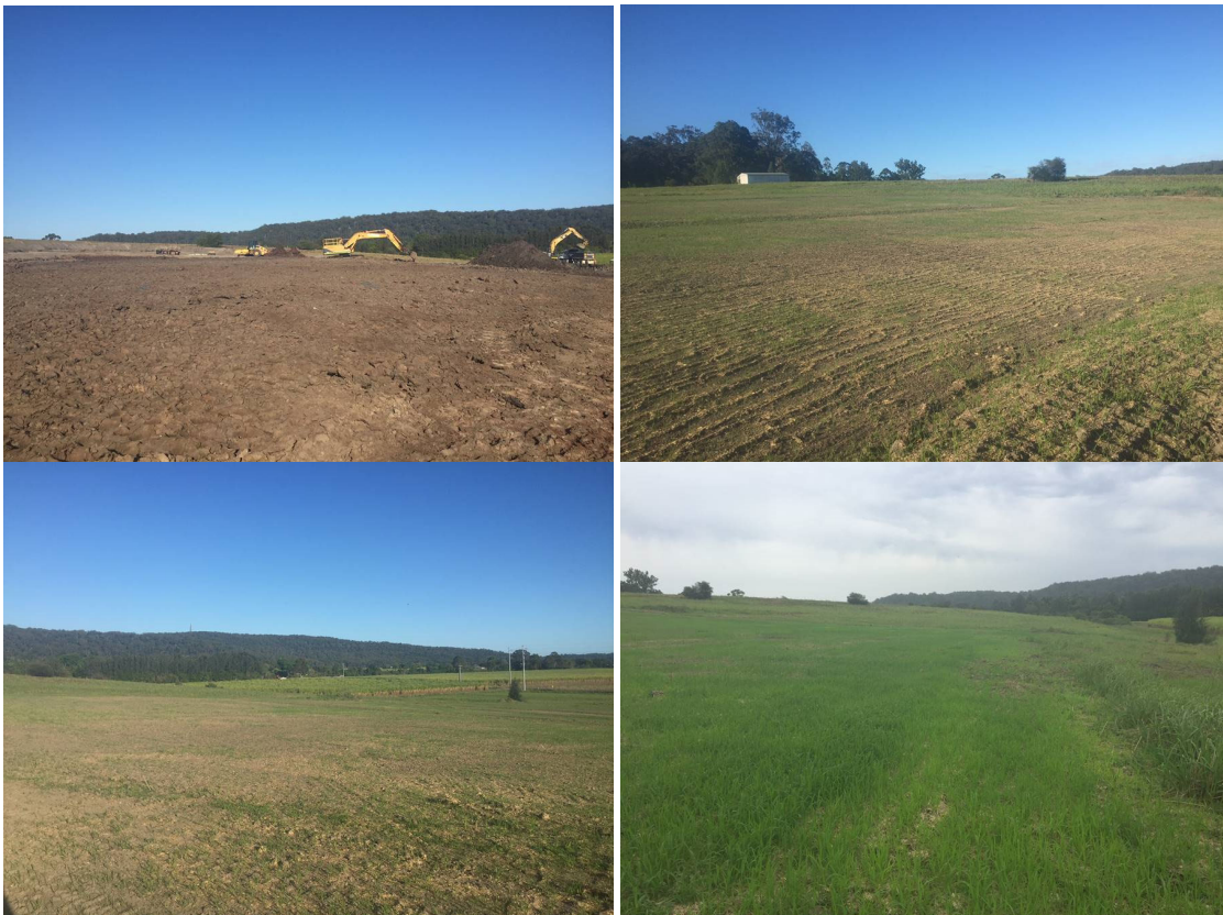
Figure 22 Earthworks – cut to fill and topsoil spreading, McIntyres Lane ancillary facility
