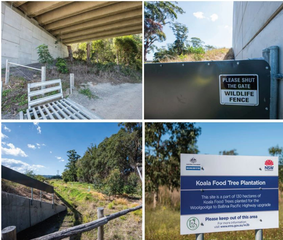
Figure 35 Wildlife protection, including Koala grids, signage, fauna furniture and culverts
