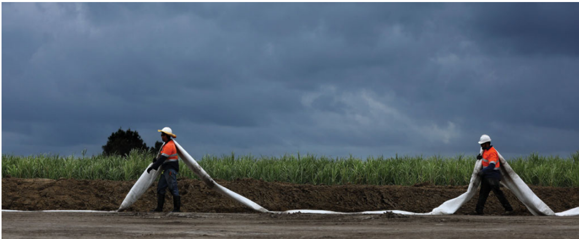
Figure 5 Workers laying out geofabric
