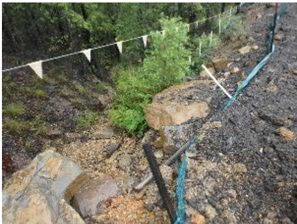
Photograph 7: Overtopping erosion control leading into a drainage line associated with in-situ Site QM-1.1 (summer 2017)
