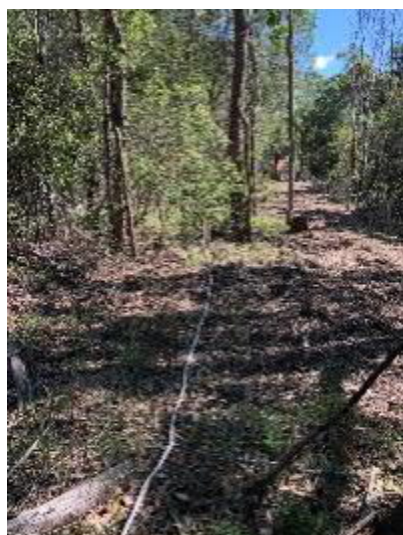
Photograph 9: Clearing and under scrubbing of Site 3.10a for fence construction
