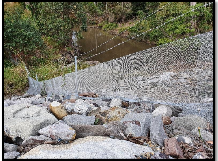
Plate 3-2. Missing frog exclusion fence at Corindi Creek on the northern abutment (left) and frog fence return facing the opposite way along with numerous holes at the bottom of the fence (right).
