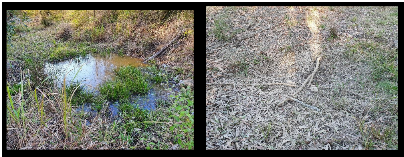
Plate 5-4. Pond inspection in late March 2020 showing ponds with (left) and without (right) water at Falconers ch. 11800.
