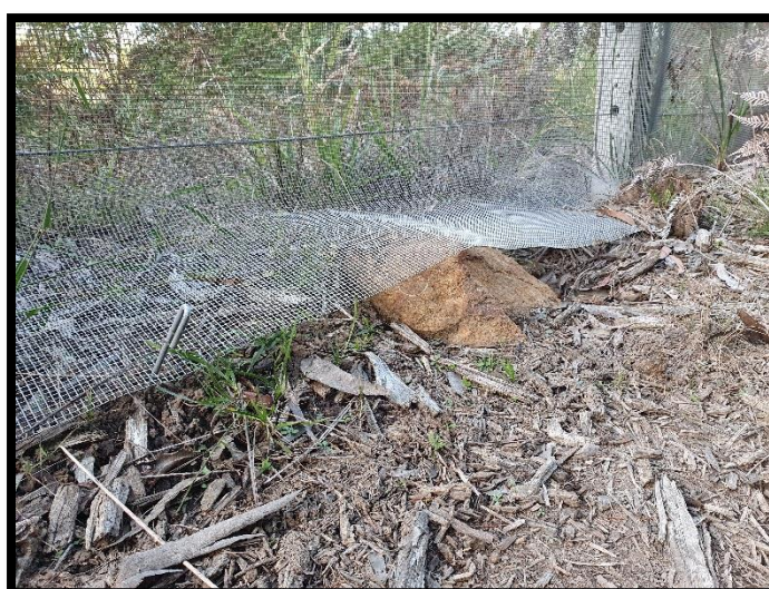
Plate 5-9. Examples of frog fence not been fixed to the ground adjacent to frog monitoring sites at Site 1A Falconers (left) and Site 2A Halfway Creek (right).
