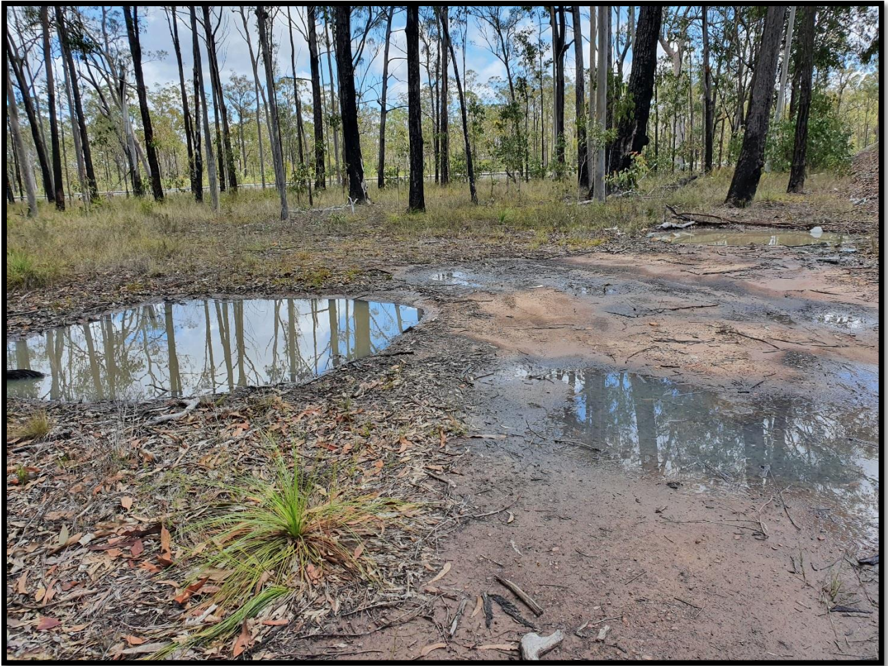
Plate 5-6. Pond inspection in mid January 2020 showing ponds at capacity following heavy rainfall.
