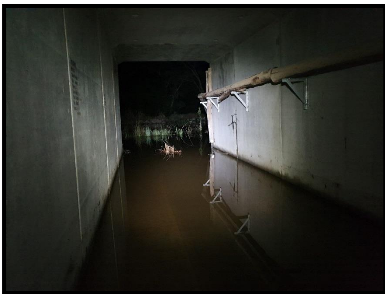
Plate 5-2. Sampling of the structure at ch.19180 on the 19 th January 2020.
