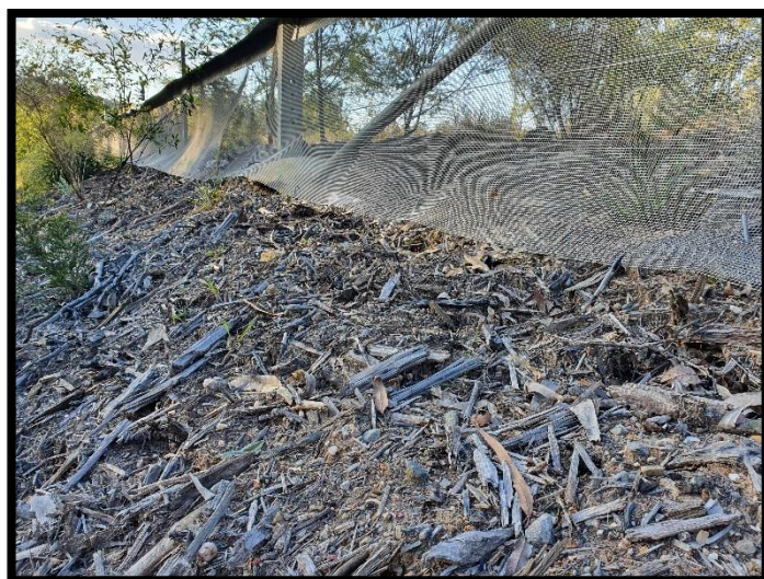
Plate 5-9. Examples of frog fence not been fixed to the ground adjacent to frog monitoring sites at Site 1A Falconers (left) and Site 2A Halfway Creek (right).
