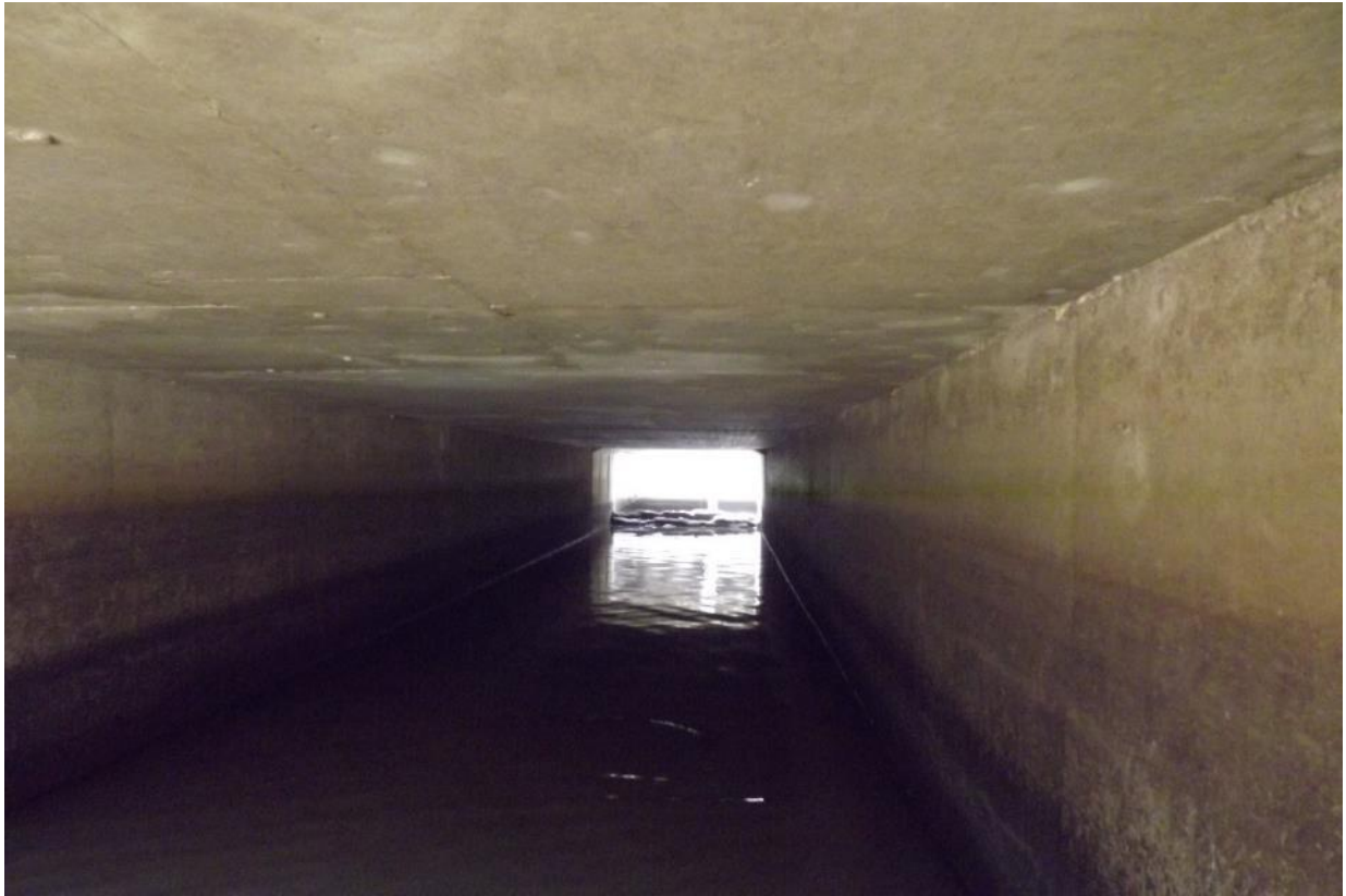
Figure 11: Looking east through Oakey Creek culvert, one of the impacted subject drainage structures along the W2B alignment showing current and previous high water levels (staining half way up culvert walls).
