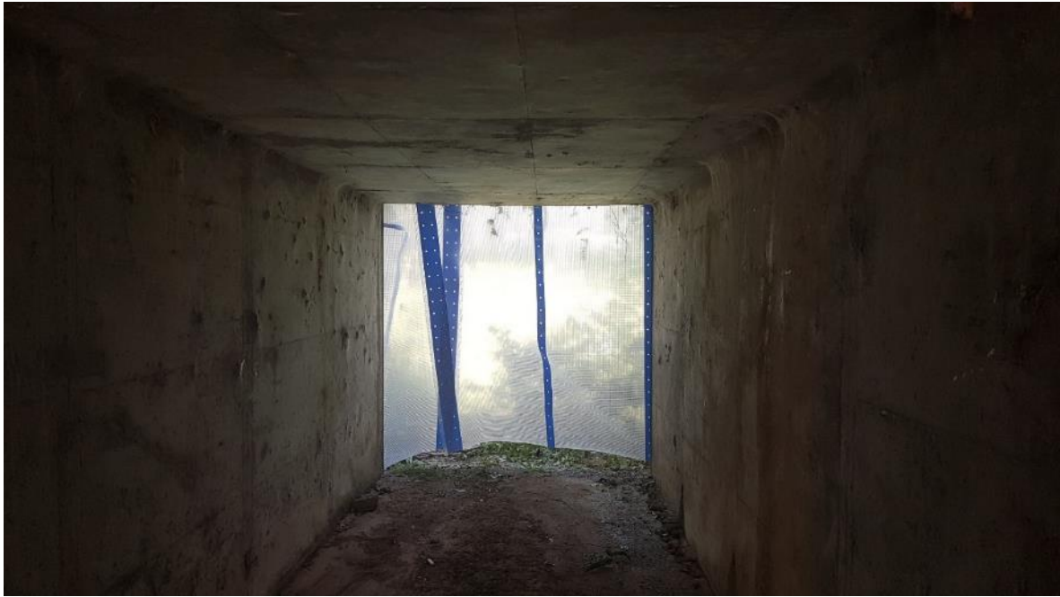
Figure 15: Internal view of exclusion device for microbats using heavy duty plastic sheeting across a culvert outlet, Devil's Pulpit tie in, Woolgoolga to Ballina Pacific Highway upgrade, April 2018.
