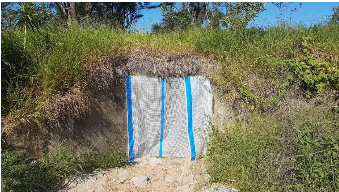
Figure 14: External exclusion for microbats using heavy duty plastic sheeting across a culvert outlet, Devil's Pulpit tie in, Woolgoolga to Ballina Pacific Highway upgrade, May 2018.
