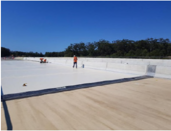
Figure 34 Waterproofing membrane application Bridge D03
