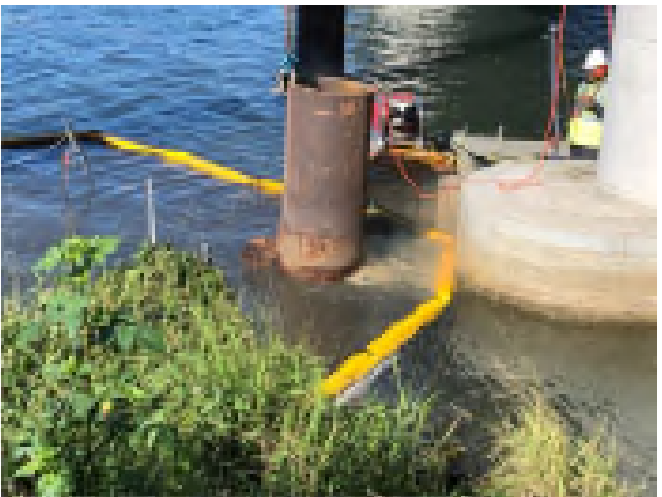
Figure 37 North side of B08 Temporary jetty pile removal with oxy-gauge cutting
