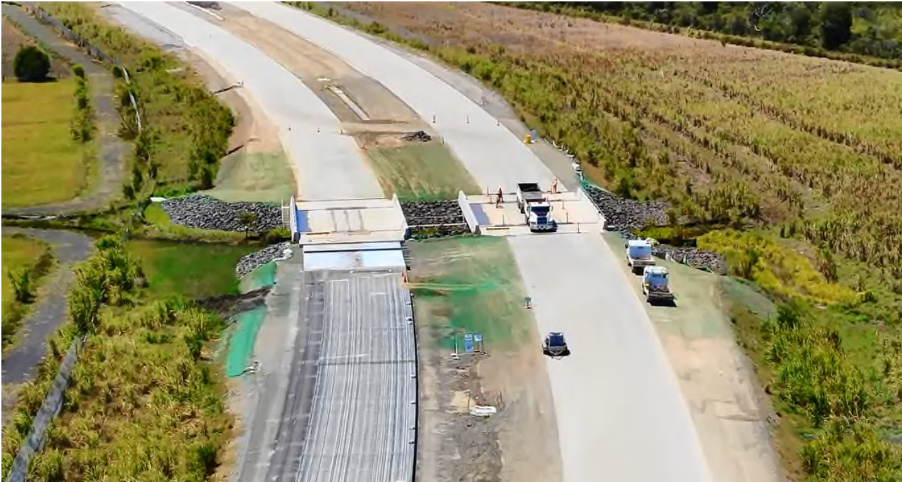
Figure 29 Removal of Bridge C52 Temporary Access and Revegetation, OPP Waterway
