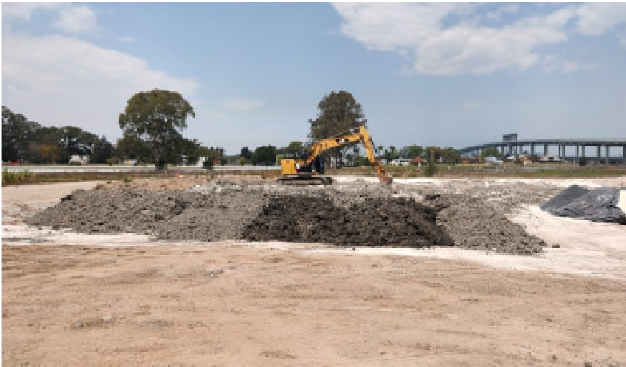
Figure 58 Treatment of acid sulfate material at Harwood ASSTA
