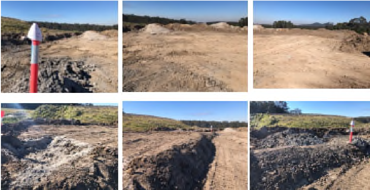
Figure 57 ASTA sump and holding bay for bridge contractor
