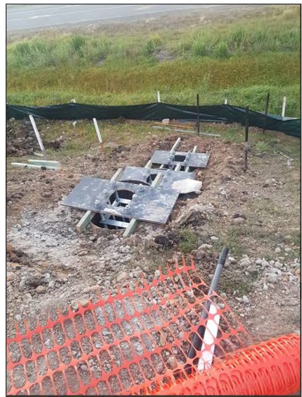
Figure 15 Installation of electrical services and structural signage footing at Harwood North in Section 5
