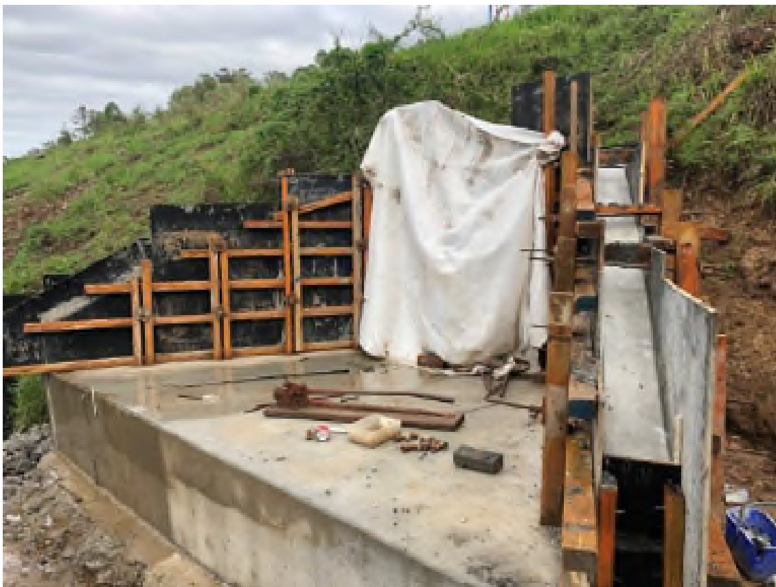
Figure 51 Microbat exclusion shroud maintained during construction of culverts
