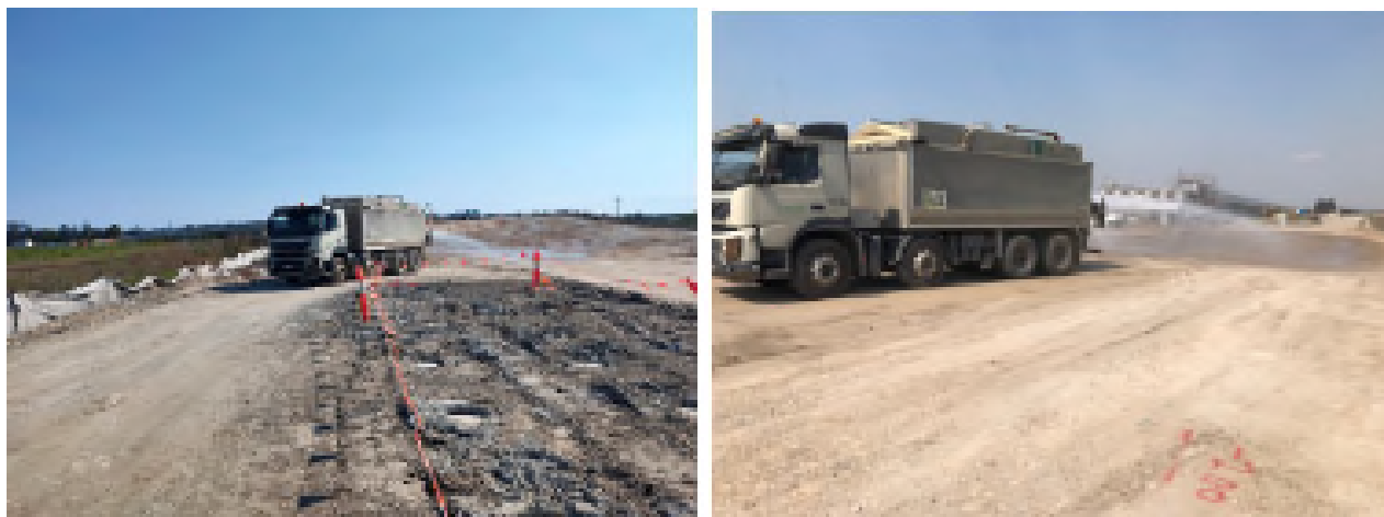
Figure 65 Watercart conducting dust suppression at Bridge B65
