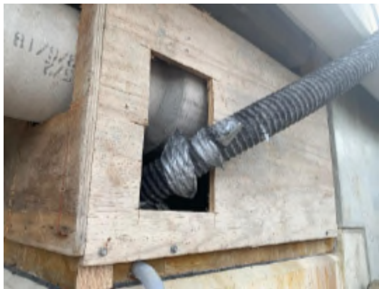
Figure 25 Encapsulation for hydro demolition works at OPP Bridge site C51; and containment of hydro demolition wastewater, preventing alkaline water reaching OPP waterways.
