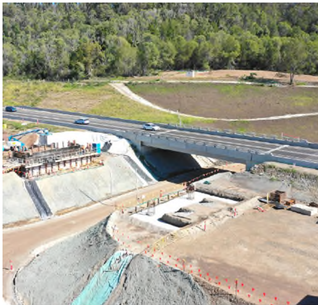
Construction continues for the new bridge over Koala Drive at Farlows Flat, Maclean
