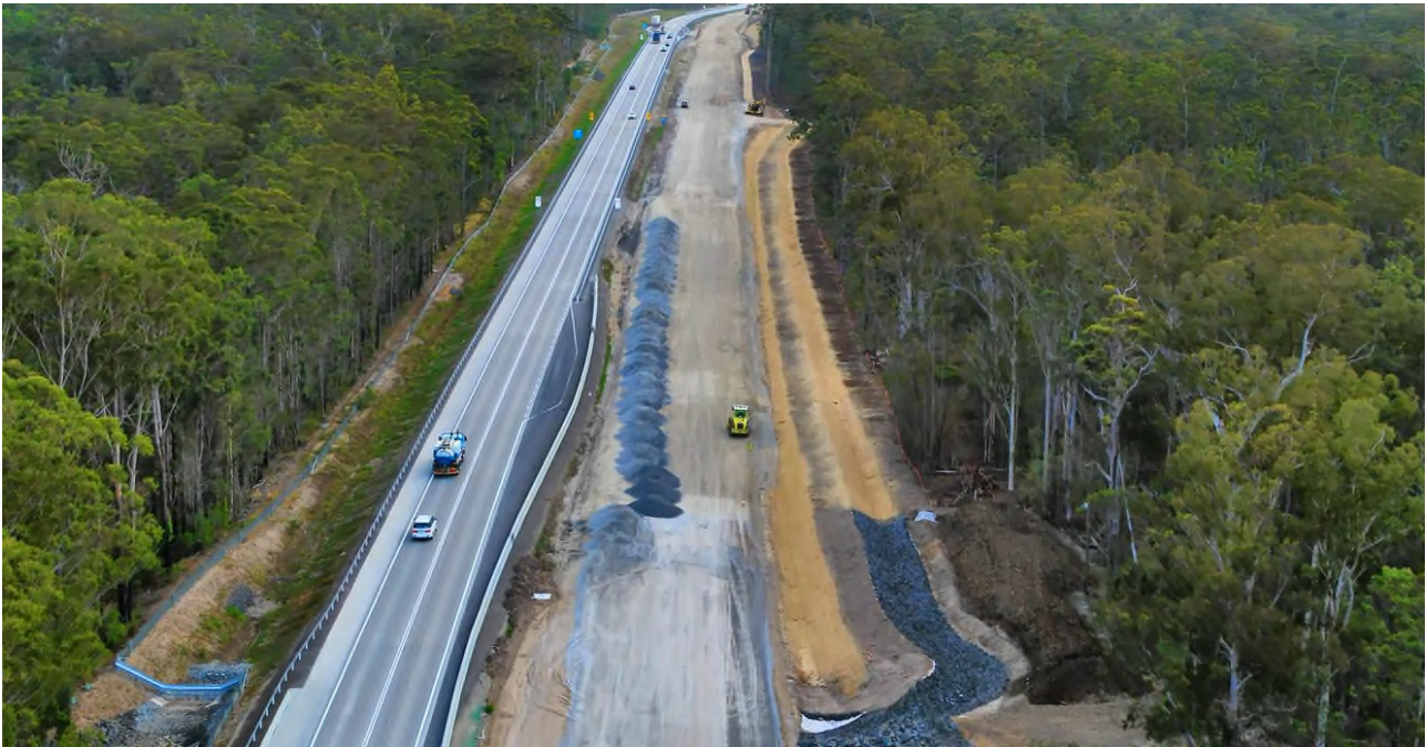
Figure 17 Progressive rehabilitation in Section 7
