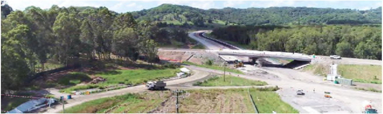
Figure 5 Aerial view of new overpass bridge at Wardell Road being built, April 2019
