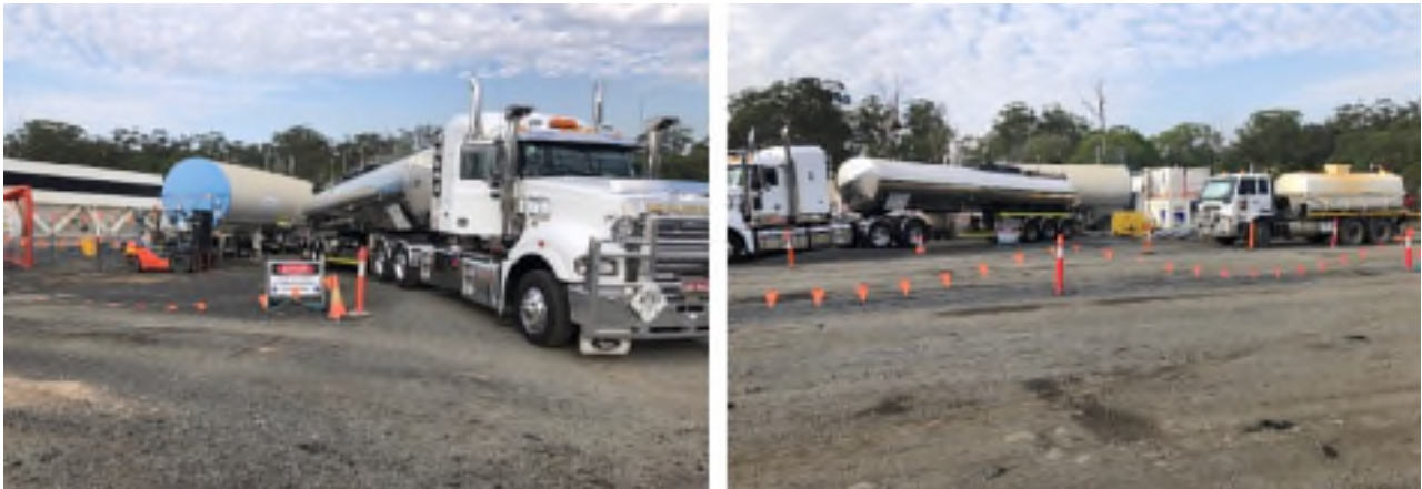
Figure 19 Exclusion zone set up during 'bitumen transfer in progress'
