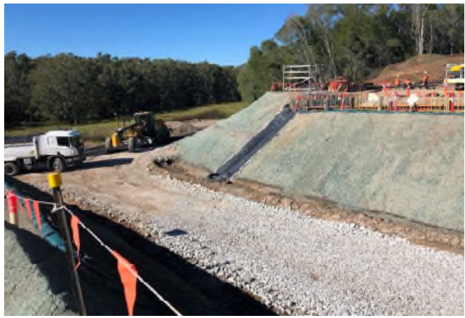
Figure 66 Rumble grids at Yamba Roundabout Figure 67 Batter chute with soilbinder Bridge B01
