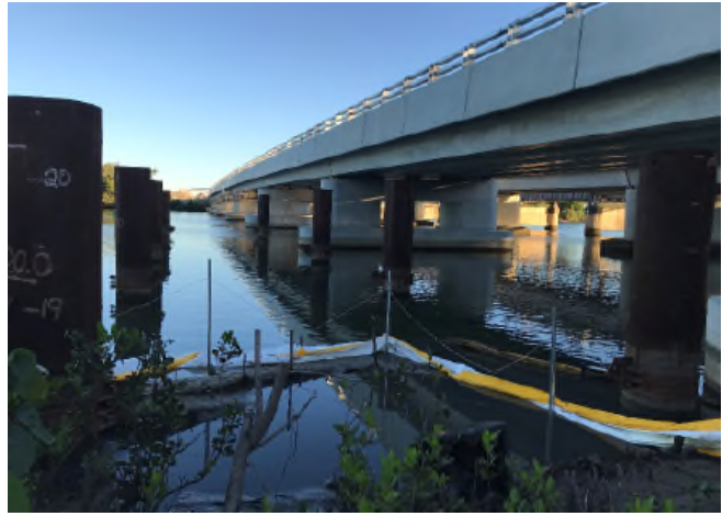
Figure 24 Waterway crossing at Bridge B67 and contingency sediment curtain maintained at B08
