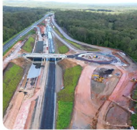
Aerial view of the Woodburn interchange looking south
