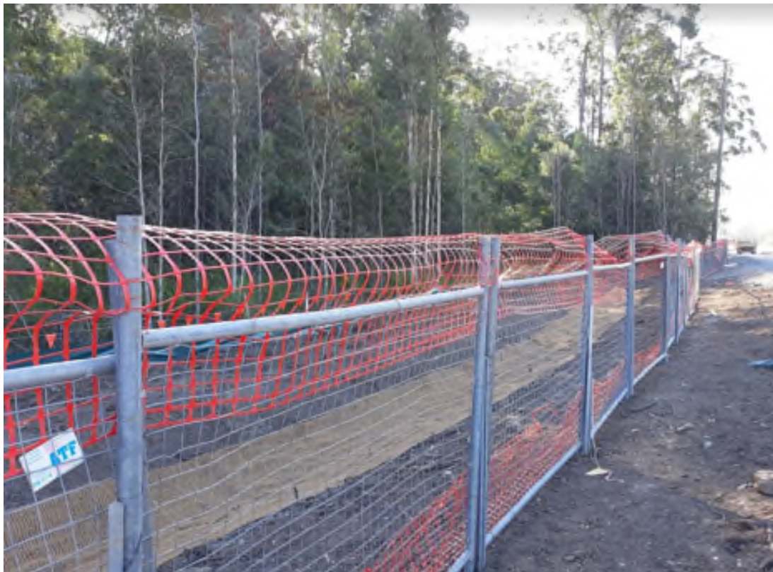
Figure 49 Installation of temporary Koala fencing during traffic switch preparation works in Section 6
