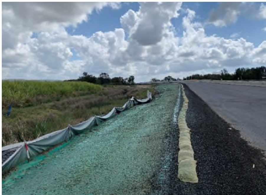
Figure 23 Sandbag edge protection and soilbinder applied to batter
