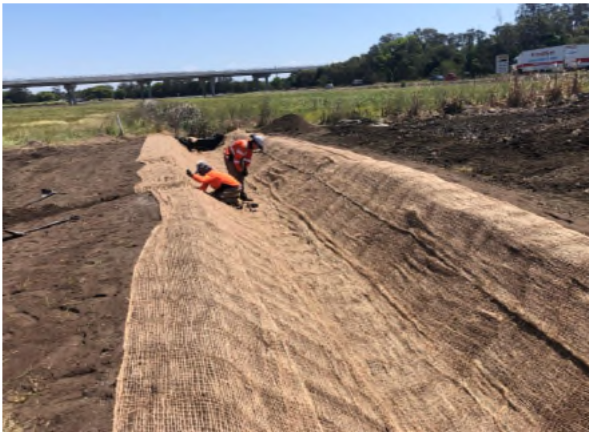
Figure 40 Drain being lined with Jute Mesh
