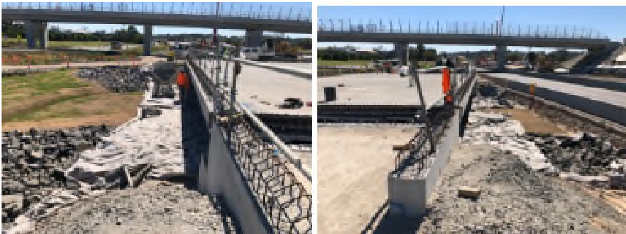
Figure 43 Bridge B67 Temporary green cutting setup over cane drains
