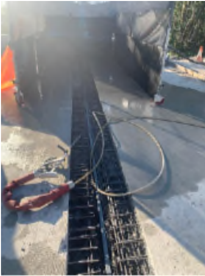
Figure 25 Encapsulation for hydro demolition works at OPP Bridge site C51; and containment of hydro demolition wastewater, preventing alkaline water reaching OPP waterways.
