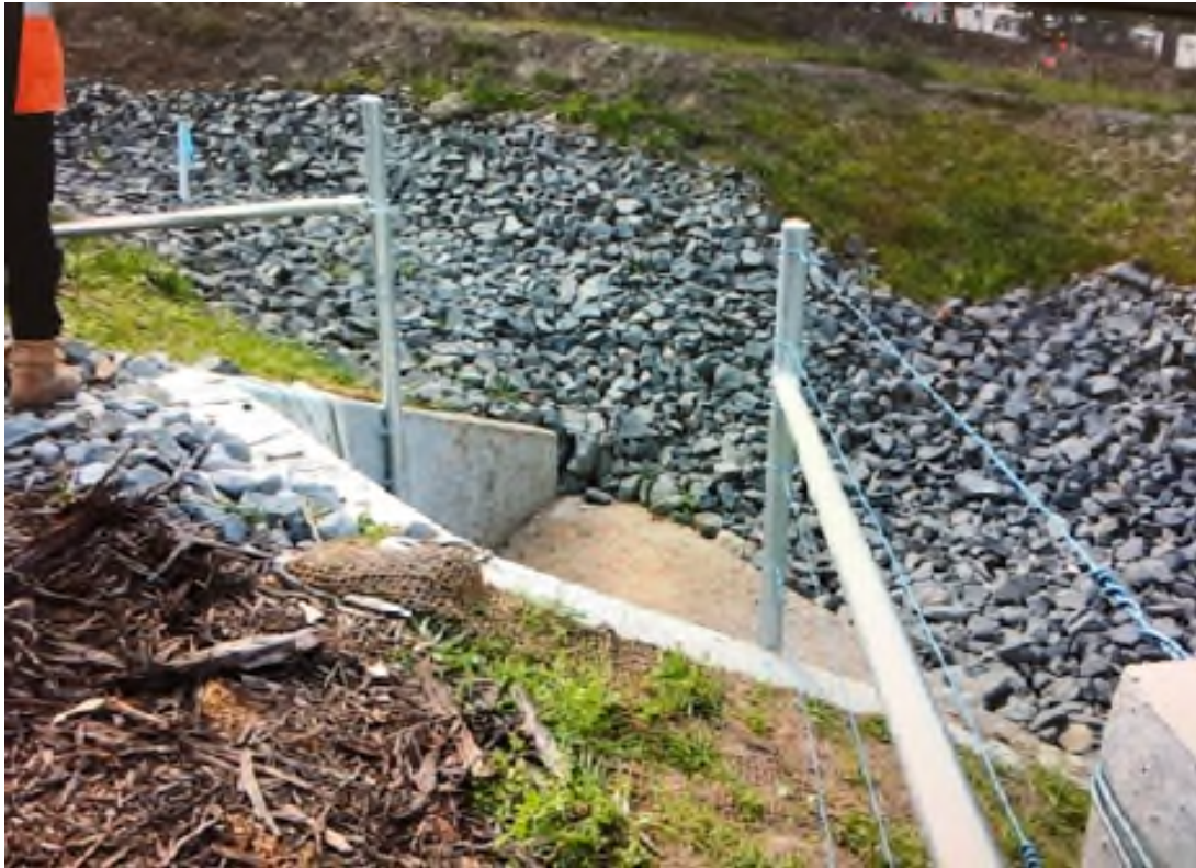
Figure 48 Drop down for fauna at Culvert CH82030
