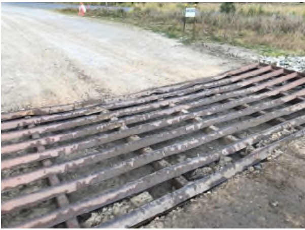
Figure 66 Rumble grids at Yamba Roundabout Figure 67 Batter chute with soilbinder Bridge B01
