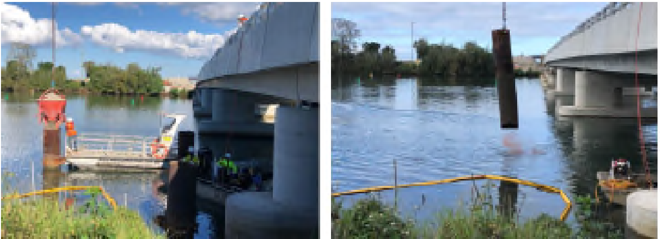
Figure 38 Loaded kibble lifted & directed over the pile by crane and the cut off section lifted over water
