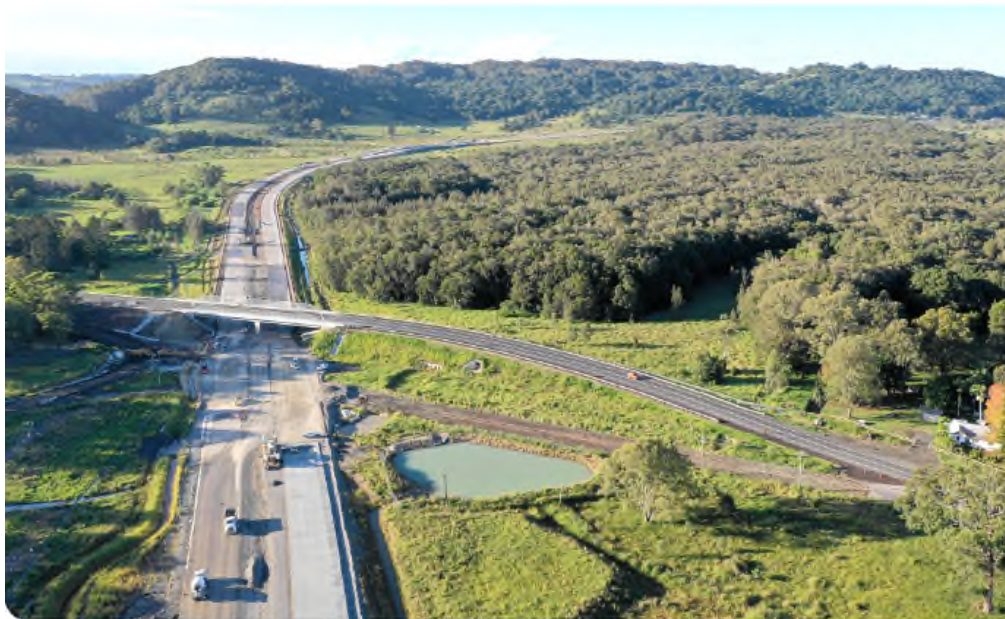
Line marking completed for the new Wardell Road overpass bridge
