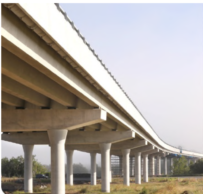
New bridge over Richmond River facing west
