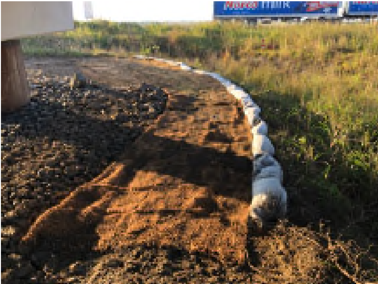
Figure 42 Bridge B64 south demonstrating temporary erosion and sediment controls, preventing turbid runoff entering cane drain.
