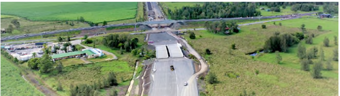
Figure 4 Woodburn-Evans Head Road overpass bridge looking north, April 2019
