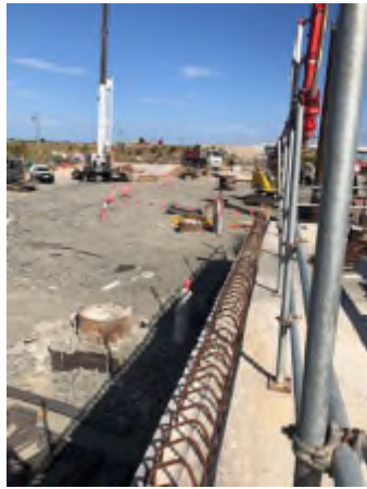
Figure 35 Bridge B08 repair works, piles being installed
