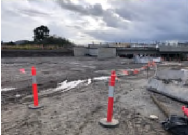
Figure 33 Bridge B08 repair works constructing piling platforms, good use of upturn geofabric and bunding at edge of platform.
