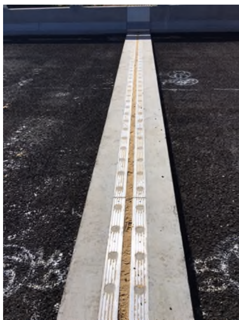
Figure 20 Sand in expansion joints prior to paving
