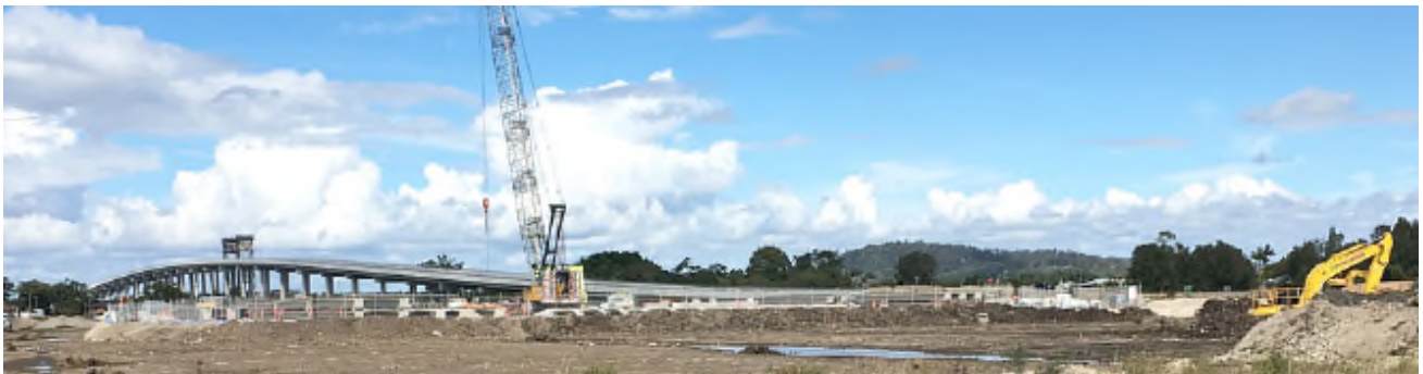
Figure 6 Site restoration works at the new Bridge over the Clarence River at Harwood, April 2019
