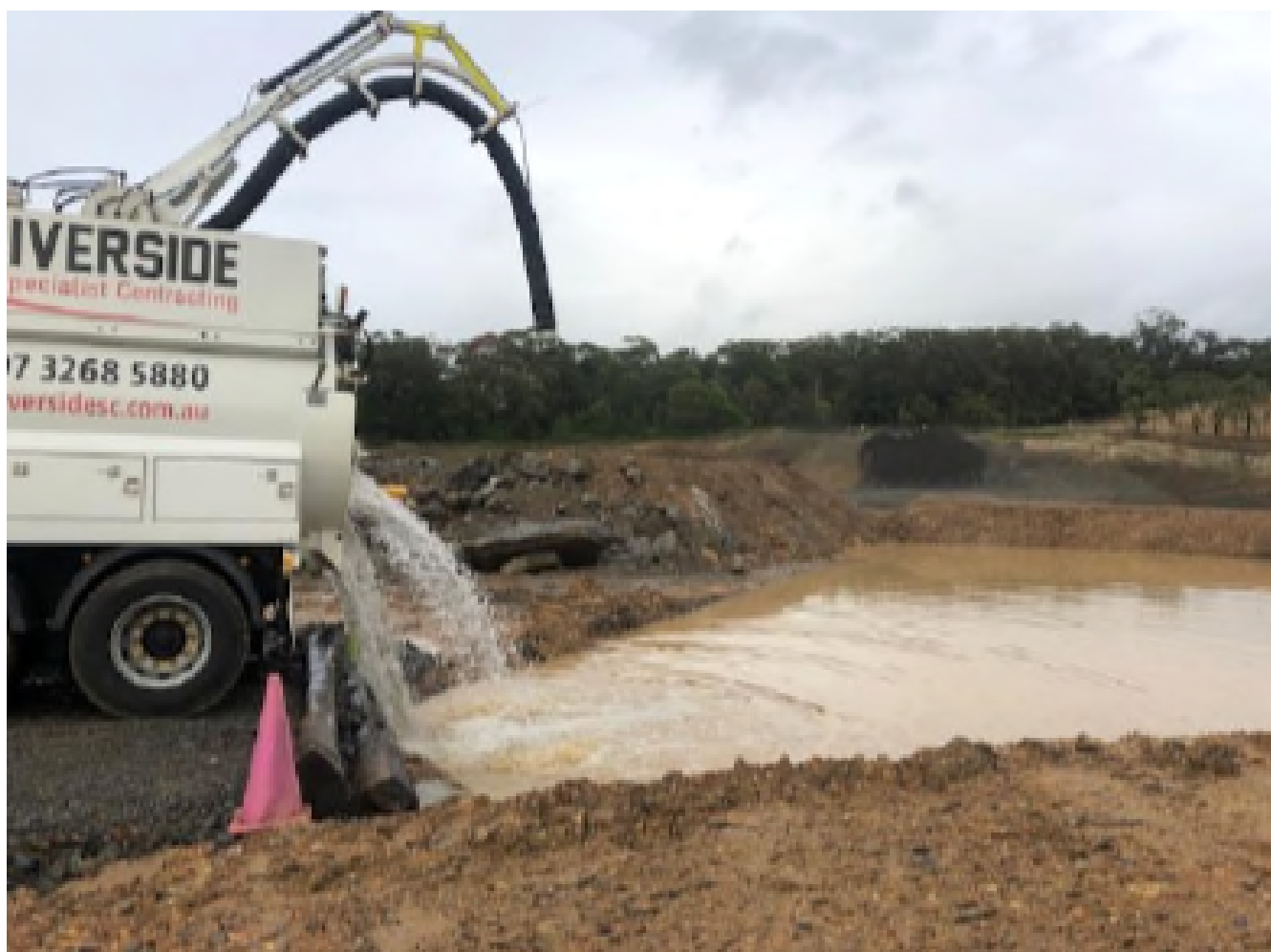
Figure 59 Hydro demolition waste water being stored and re-used for dust suppression
