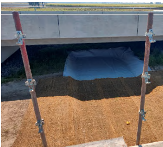
Figure 41 Jute mesh installation & ground cover at Bridge B67; and jute mesh and geofabric protection for swale drain at Bridge B68
