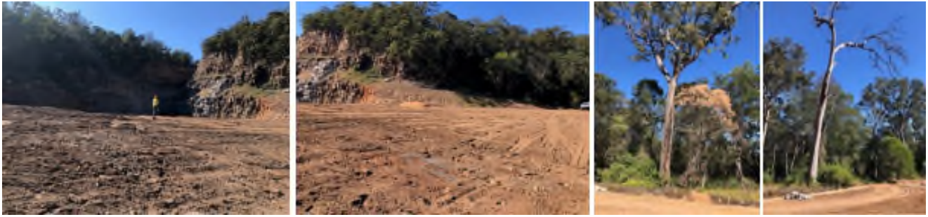
Figure 18 Tyndale Borrow site rehabilitation, noting habitat trees in tact
