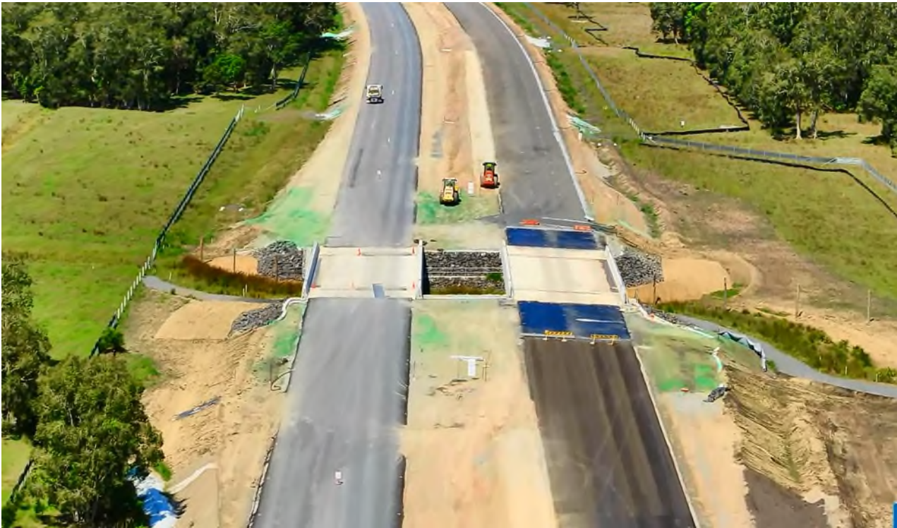
Figure 30 Removal of Bridge C53 Temporary Access and Revegetation
