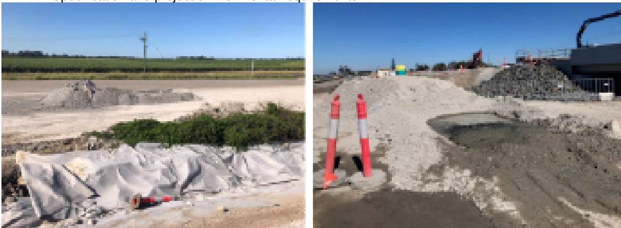
Figure 52 Bridge B56 & B55 concrete washout bay / reuse of concrete with general fill.
