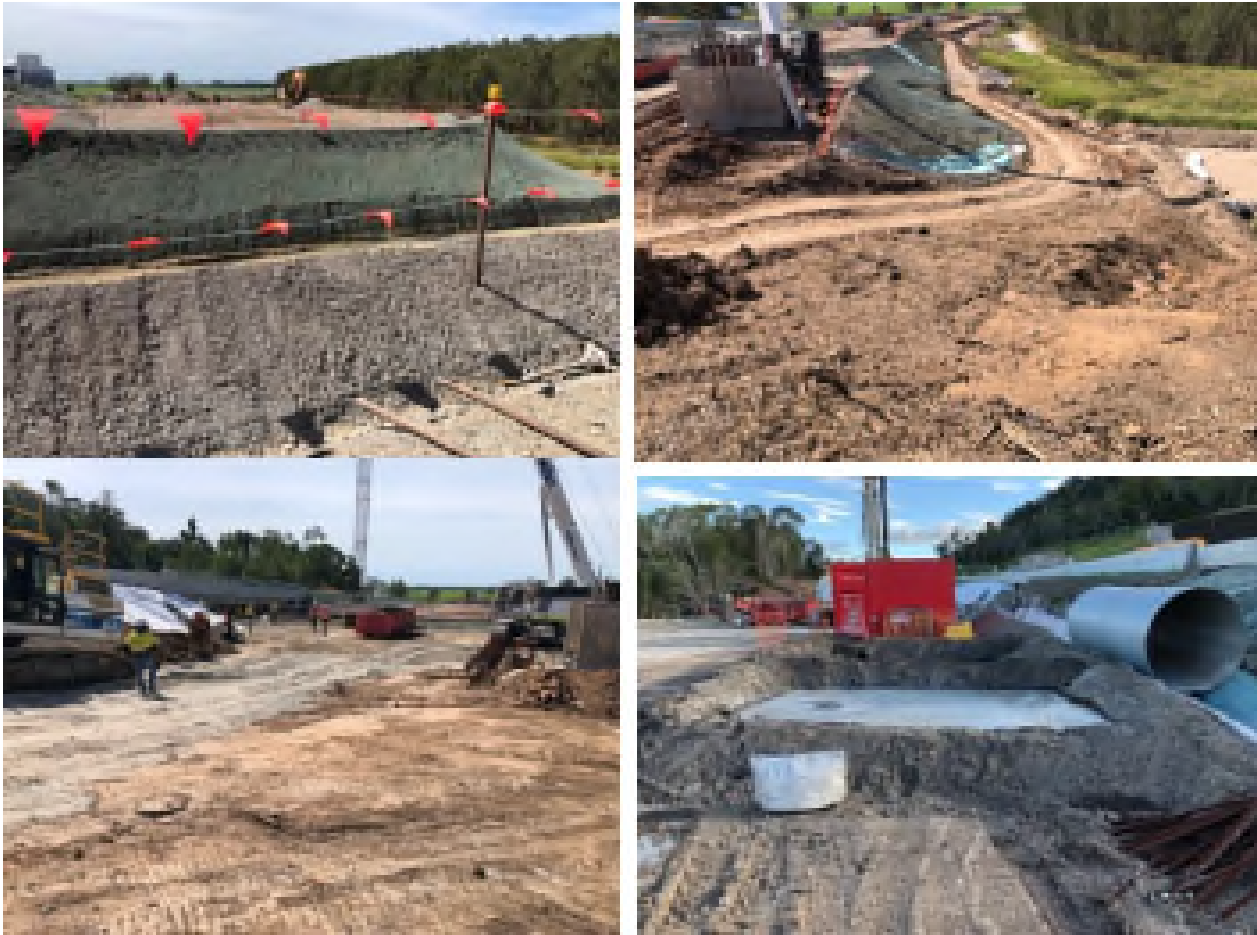
Figure 22 Bridge B01 - soil binder on abutments, earth berms, lined temporary batter chutes and batters, and lined dirty diversion drain
