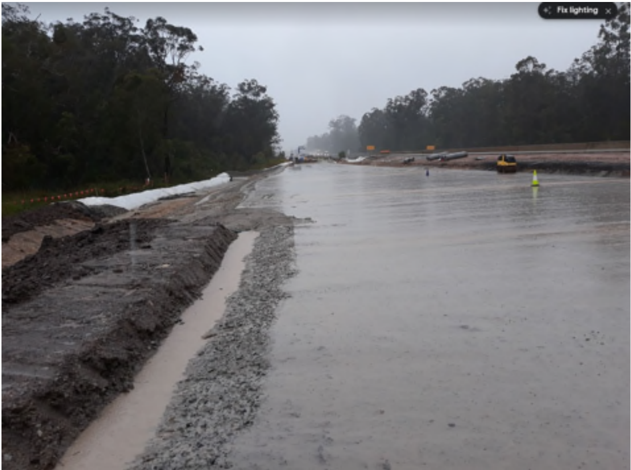
Figure 27 Runoff from works directed via a reverse grade drain towards 90 th percentile rainfall event, oversized basin in OPP Water Management Area Section 6.
