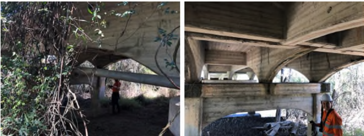
Figure 69 Serpentine Channel Bridge Flying-Fox Monitoring
