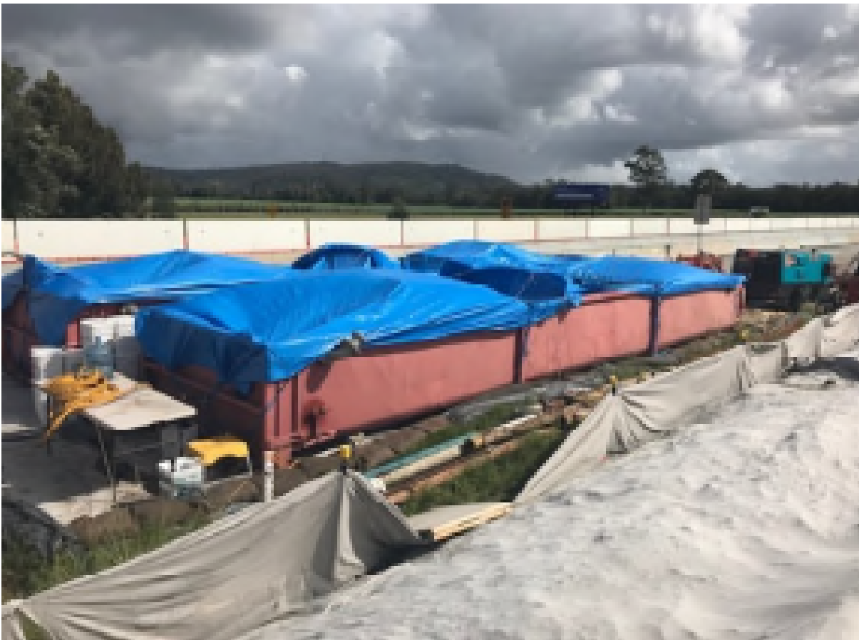
Figure 31 Covering polymer tanks prior to rainfall at Bridge B68
