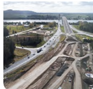
Earthwork progressing at the Yamba interchange
