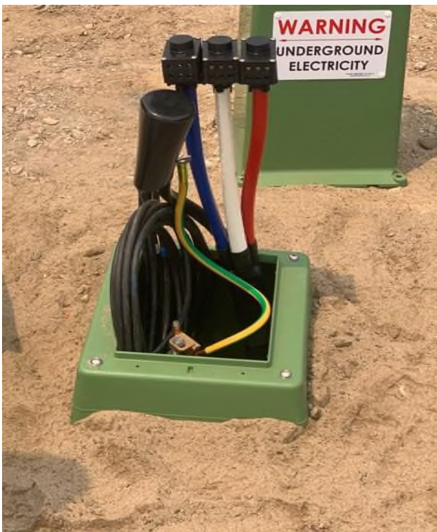
Figure 15 Installation of electrical services and structural signage footing at Harwood North in Section 5
