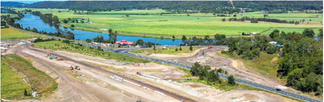
Figure 2 Future Maclean Interchange eastern roundabout progress following release of soft soil sites, April 2019
