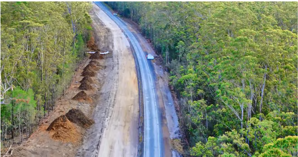
Figure 54 Mulch Reuse on Site in Section 7
