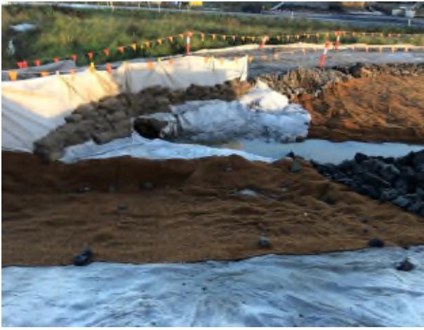
Figure 24 Waterway crossing at Bridge B67 and contingency sediment curtain maintained at B08
