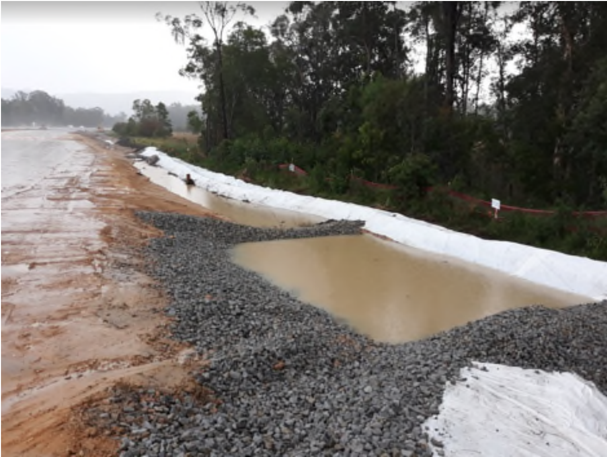
Figure 26 Controls functioning effectively north of bridge 10 Tabbimoble Creek OPP Water Management Area
