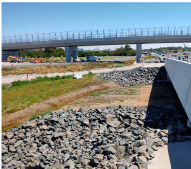
Figure 41 Jute mesh installation & ground cover at Bridge B67; and jute mesh and geofabric protection for swale drain at Bridge B68
