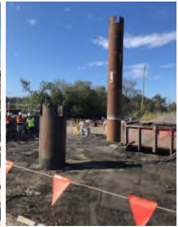
Figure 35 Bridge B08 repair works, piles being installed
