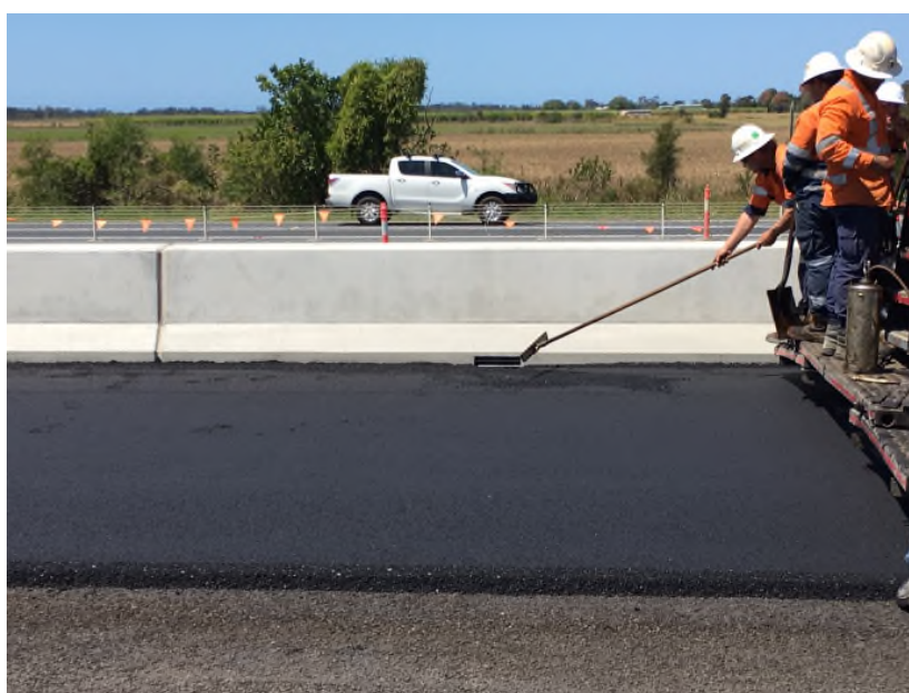
Figure 21 Asphaltting in Section 5
