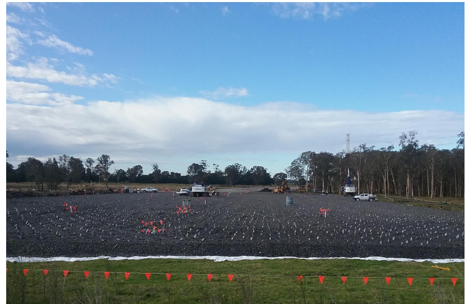
Soft soil work – foundation rock being placed
