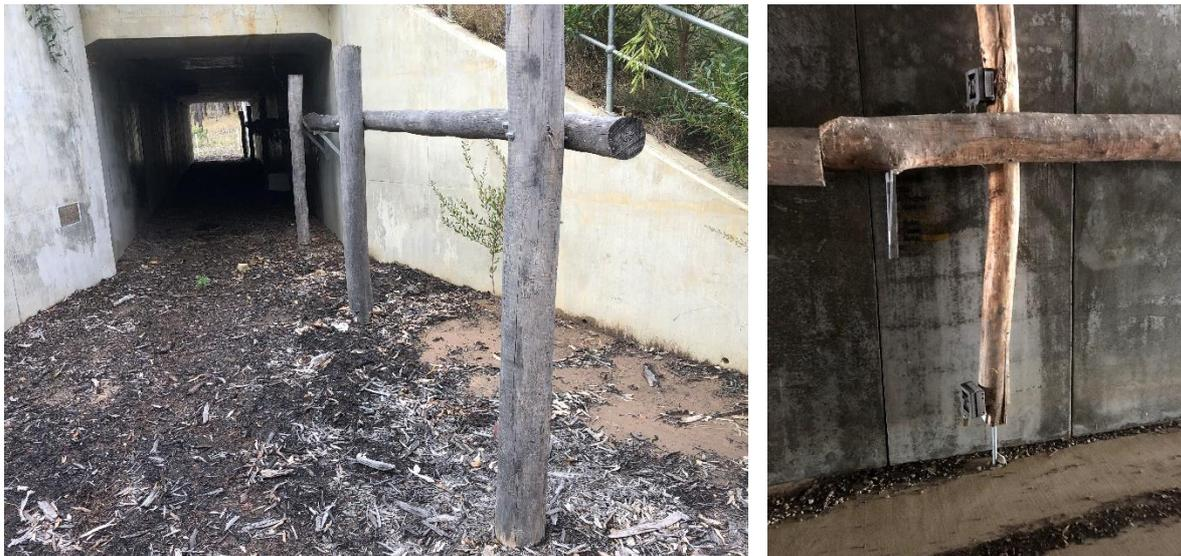
**Plate 1:** All monitored box culverts contained fauna furniture and some featured mulch spread over the concrete floor (left). Cameras were installed on the center post within each culvert – one viewing along the rail and the other along the floor (right).
