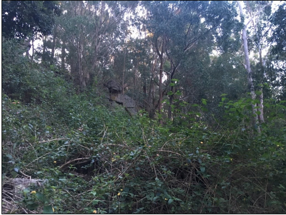
Figure 3: The general location of the sandstone escarpment, severely overgrown
