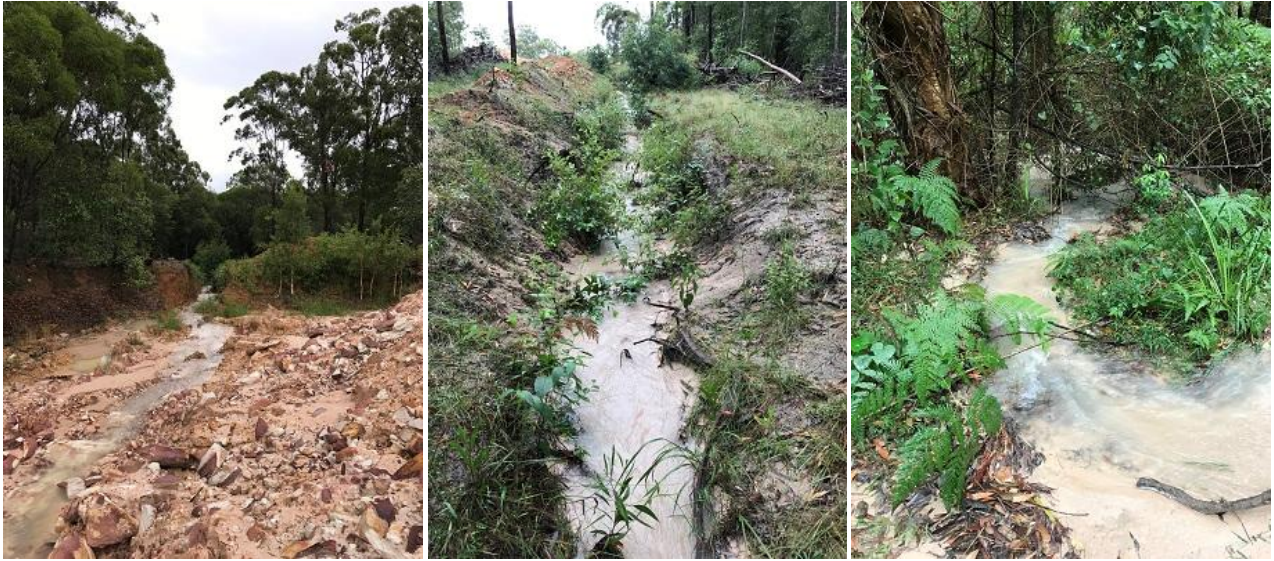
Photo 5: Uncontrolled water flows from the eastern pit into adjacent area of native vegetation and drainage channel
