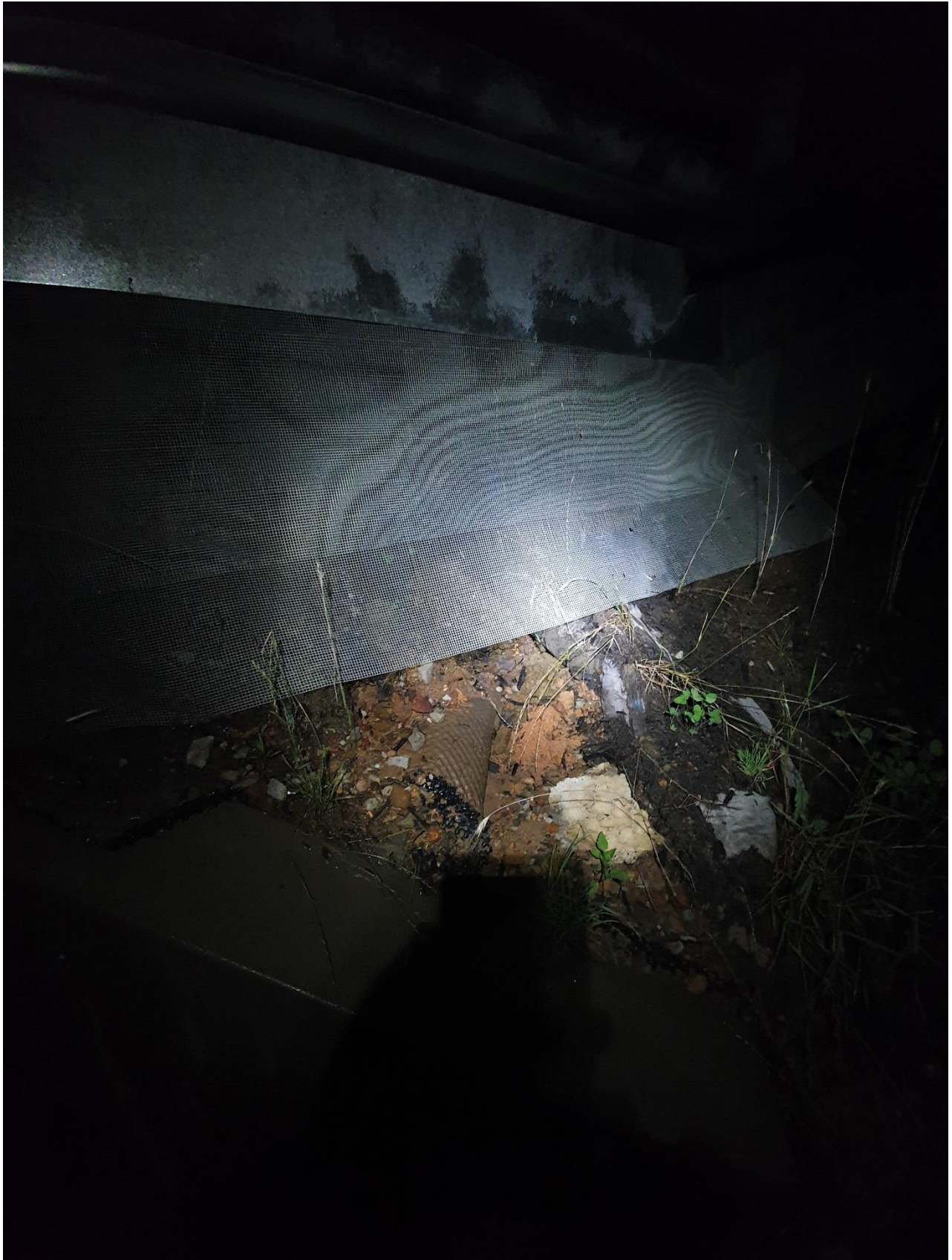
Plate 4-12. Example of a breach point at a monitored connectivity structure: Site 7A ch. 37330 inlet side of wing wall.
