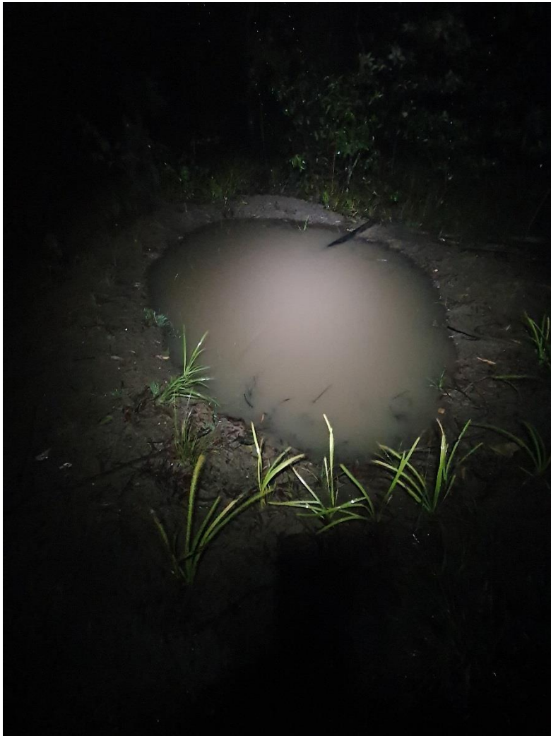
Plate 4-9. Constructed ponds at Tyndale Site 8A (ch.37330) in mid December 2020.
