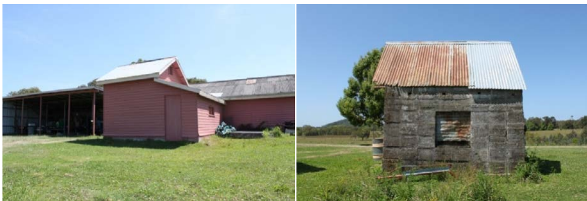
Photo 4: Item 26 Maloney Property (Buttery/Creamery and Dairy), Broadwater
