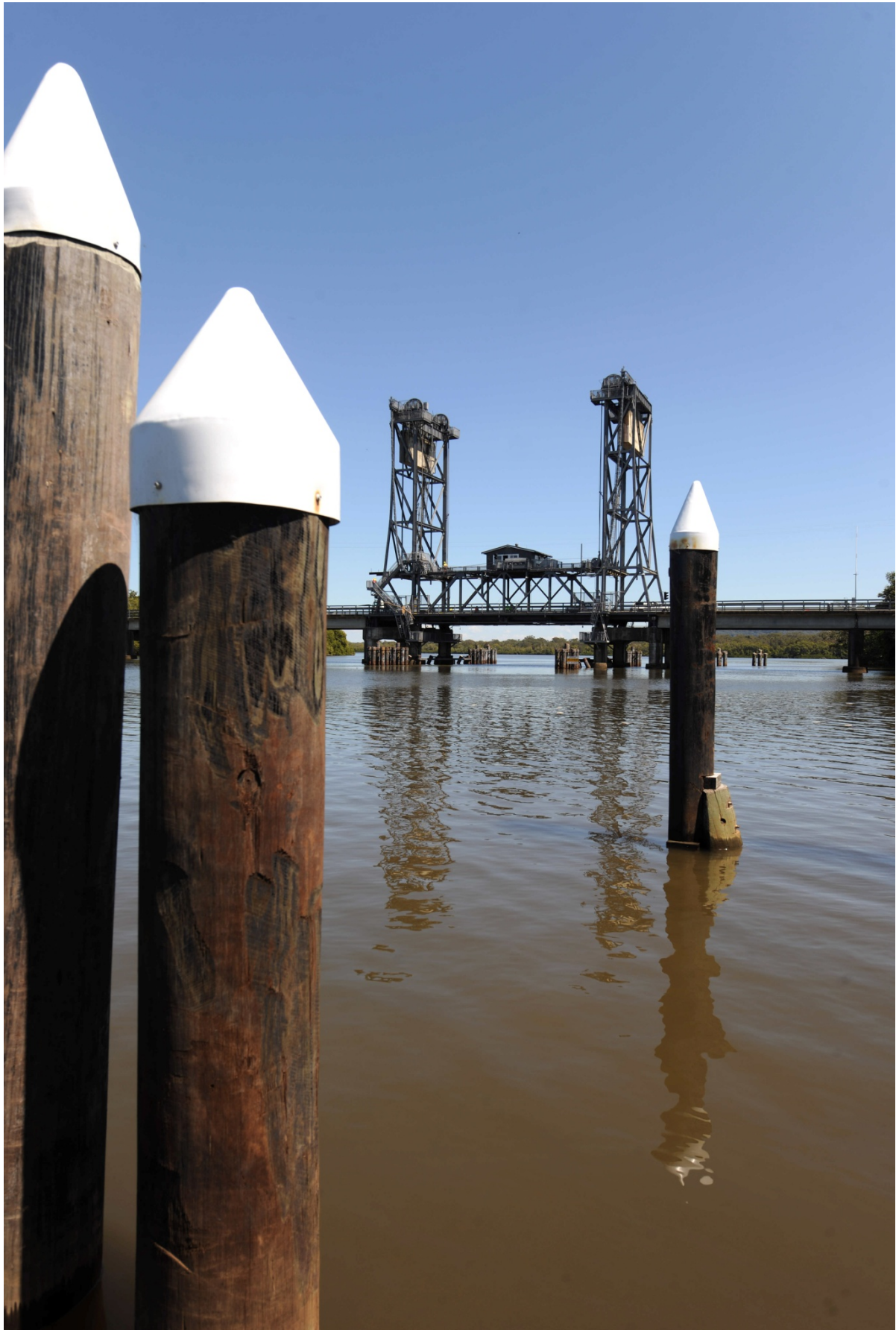
Photo 10: Wardell bridge over Richmond River
