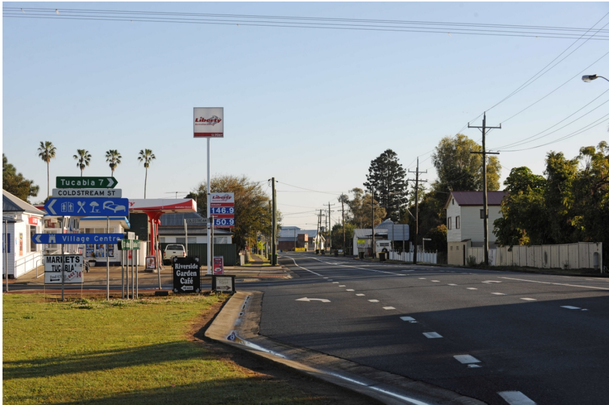
Photo 3: View of Pacific Highway through Ulmarra village
