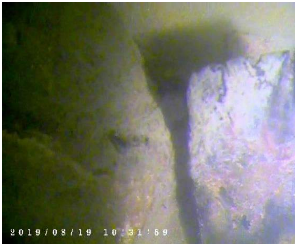
Figure 320: Timber plank 01-190819 abutting rock armour north side Hawkesbury River, scarph joint visible at top of timber. Diver facing north. (Video: WBRP Rock Armour run 001, still image taken at 00:08).
