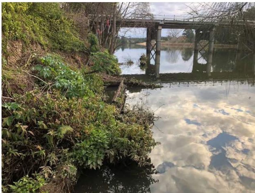
Figure 65: Overhanging vegetation and the river water level covering the riverbank wharf features. Water and deck beam visible centre of image, further wharf remains obscured by vegetation at bottom centre of image. (Image taken 16th July 2018, Cosmos Archaeology).
