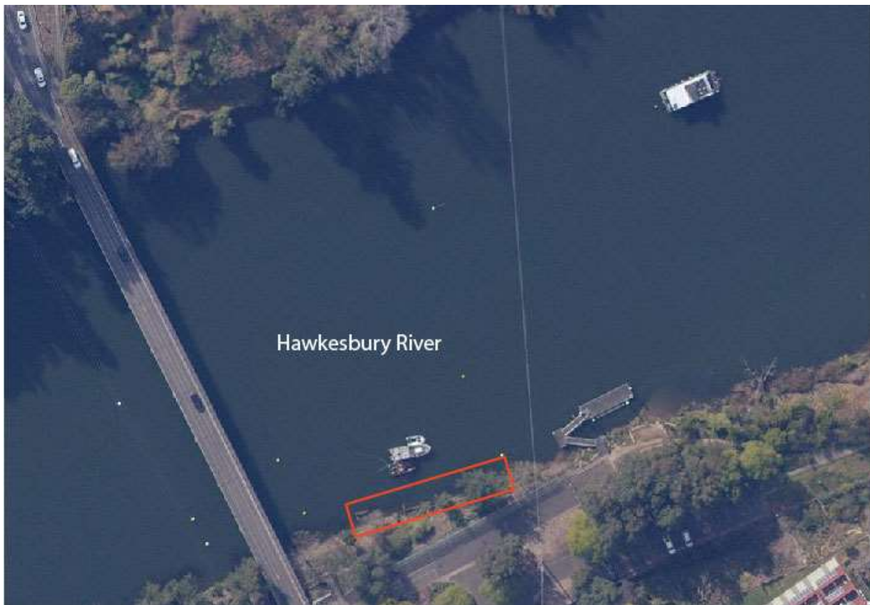
Figure 89: The wharf survey study area (red rectangle) on the southern side of the Hawkesbury River. The yellow buoys around the dive marked out the designated work area for the excavation. (Image source: SixMaps).
