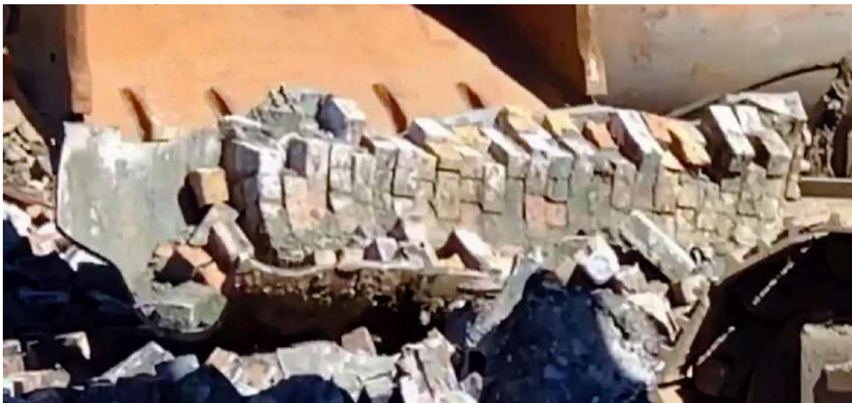
Figure 164: Demolished iron pier from 1874 Windsor Bridge showing longitudinal view of layered internal brickwork (photograph by Paul Caleo, April 2020). 269
