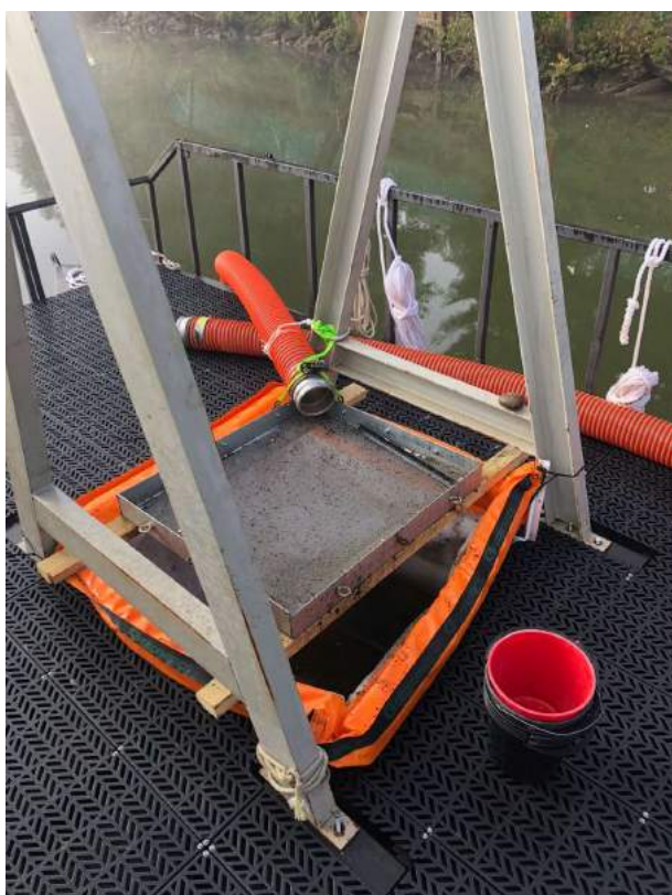
Figure 69: Set up of the sieve, silt curtain and dredge for sediment on the riverbed.
