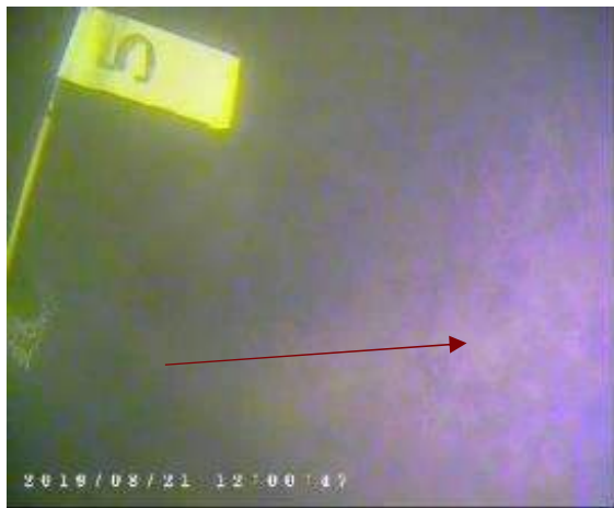
Figure 313: uncovered geofabric to the right of the transect line at the 5 m marker. (Video: WBRP Rock Armour run 005, still image taken at 01:06)
