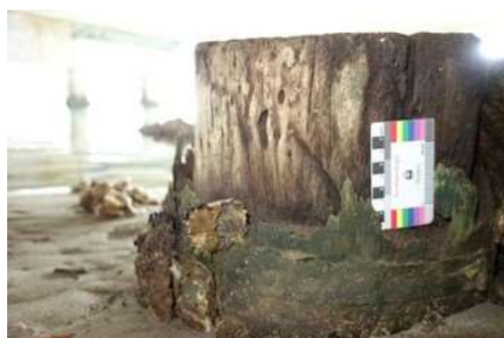
Figure 278: Copper sheathed pile stump of the former Burrill Lake Bridge.
