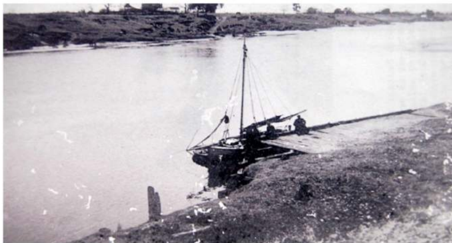
Figure 33: Windsor wharf, ca. 1920s, missing superstructure at upstream end and remnant pile stump. 120
