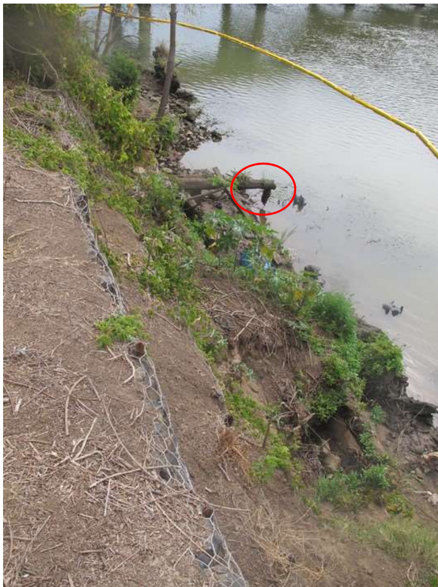
Figure 297: The timber waler (AWF6/4) associated with the 1882 wharf (Phase 3) that was to be cut as to not further strain the remaining structure (red circle).
