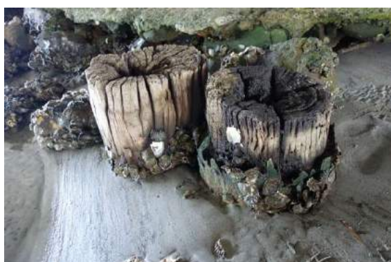
Figure 277: Timber pile stumps of the former Burrill Lake Bridge. The stump on right of image is copper sheathed. 283
