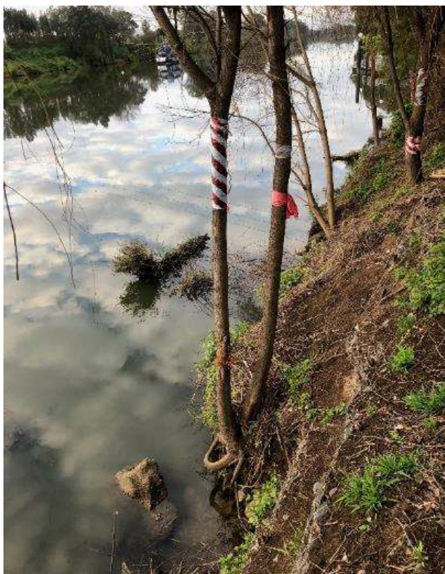
Figure 66: The steep slope and gradient of the riverbank. Top of gabion baskets are indicated with red arrows. Image taken 16th July 2018, Cosmos Archaeology).
