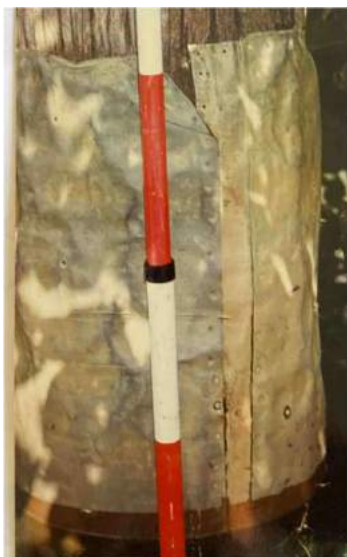
Figure 279: Copper sheathed pile at Government Wharf, Coraki, Richmond River. 284 Scale in 200 mm increments.
