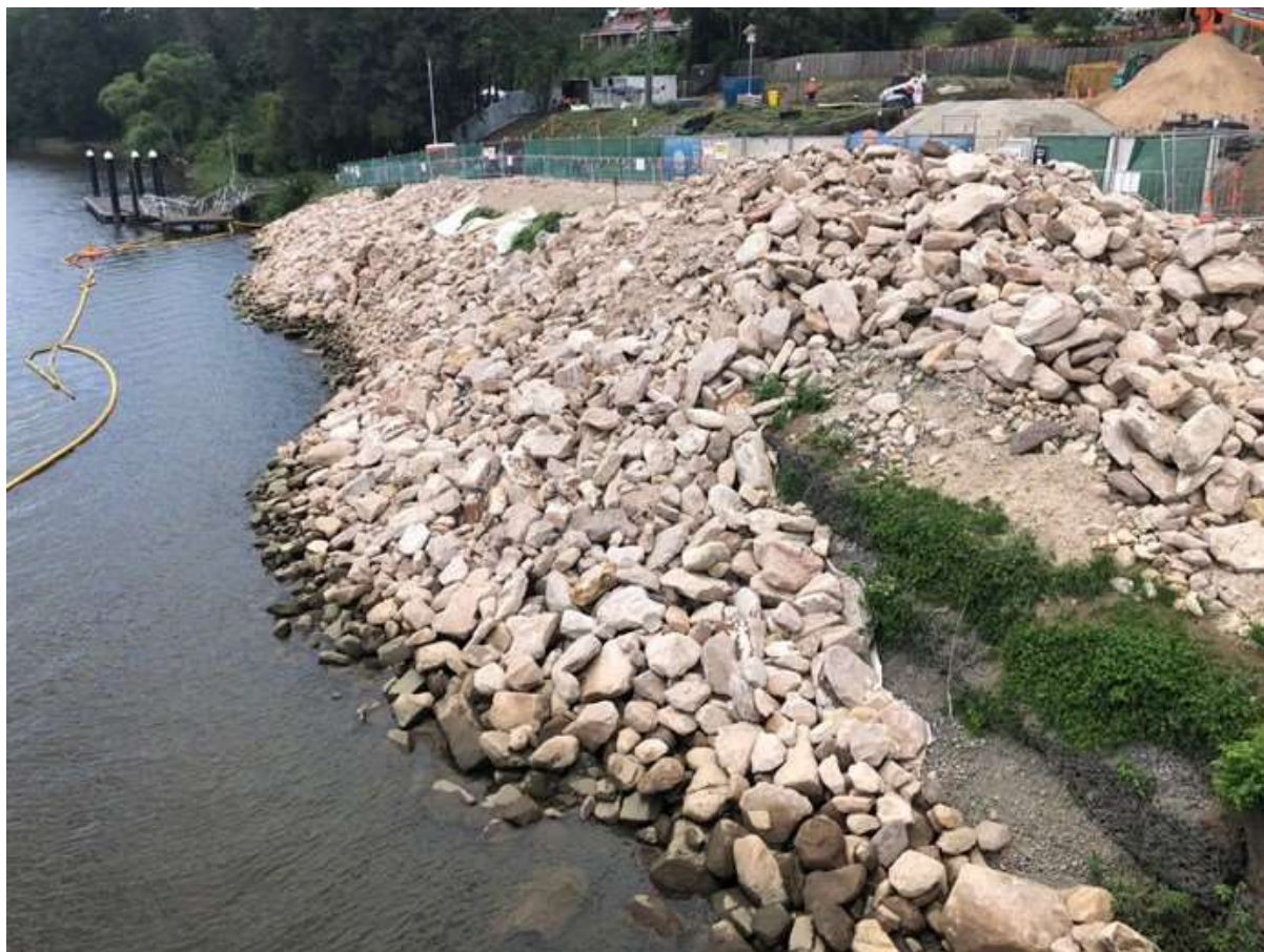
Figure 302: An in progress shot of the rock armour scour protection being laid. Taken 14th December 2018. Looking east. The site of the former Windsor Wharf is protected under the scour protection.
