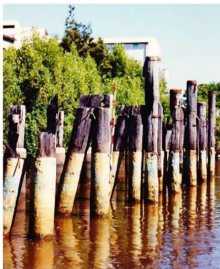
Figure 280: Piles with sheathing, Sugar Wharf, Broadwater on Richmond River. 285
