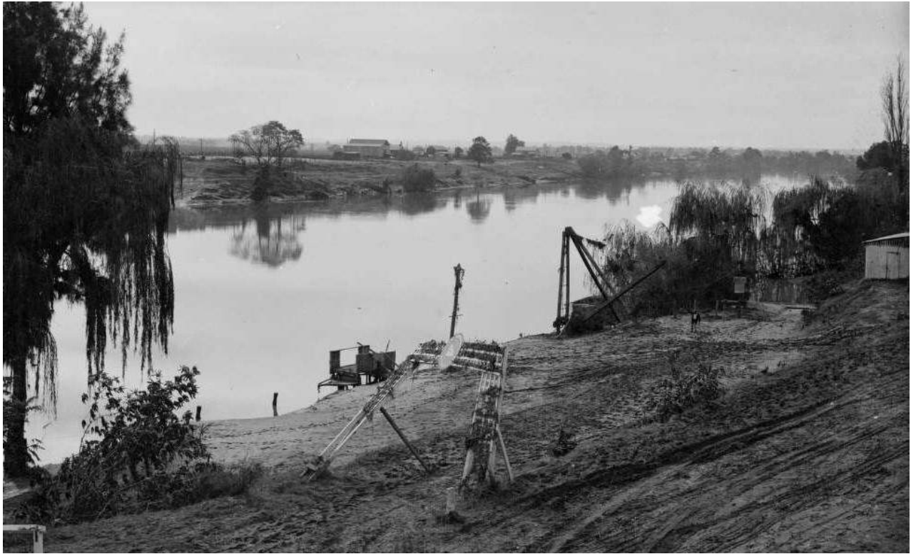
Figure 36: 1949 photograph of Windsor wharf reserve after a flood – showing pile stumps as the only visible surviving remnants of the wharf. 125
