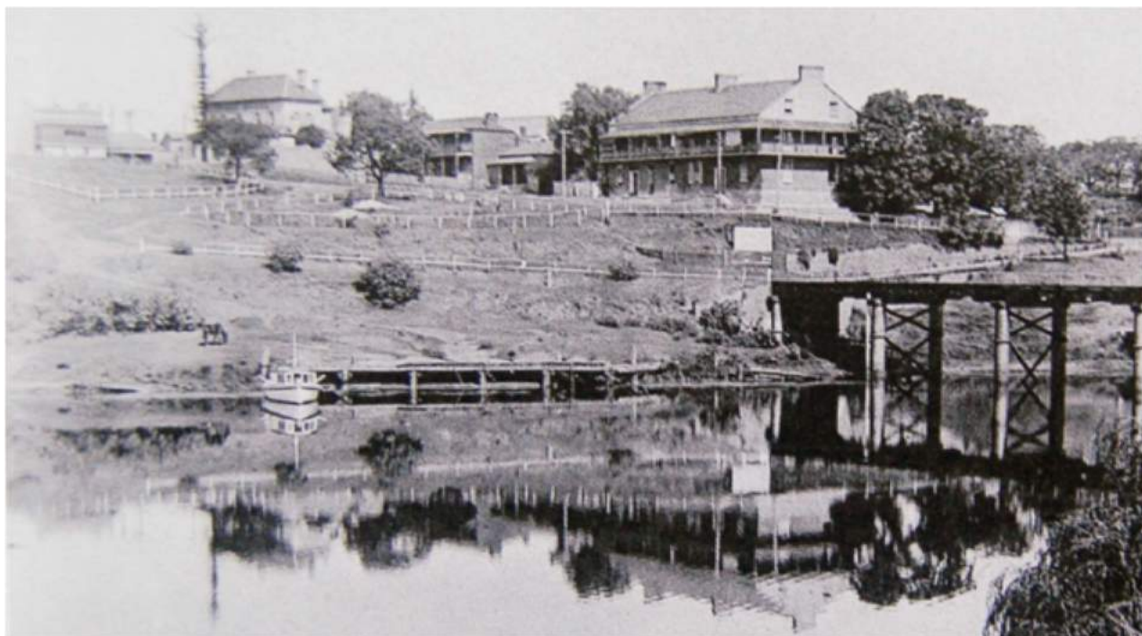
Figure 29: Windsor wharf, ca. late 1890s – showing what appears to be some deterioration of superstructure elements at the upstream end. 114
