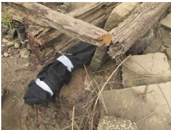
Figure 300: Timber AWF 6/4 wrapped in geofabric materials and placed underneath remaining structure of feature 6. Visible is the junction of 6/4 and 6/1 where the timber was cut back to (red circle).
