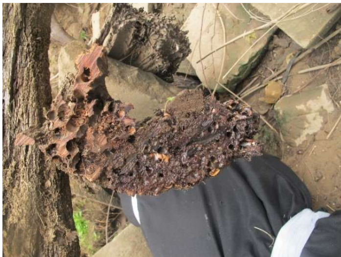
Figure 301: A section view of the remaining piece of AWF6/4. Timber piece severely damaged from marine borer activity.
