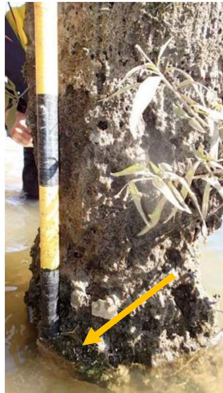
Figure 122: Only small sections of sheathing survive on the western side of AWF7, indicated by orange arrow. Scale in 100 mm increments.
