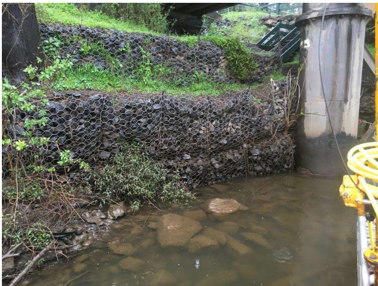
Figure 64: Gabion baskets shoring up the riverbank and rock armour in the shallow water laid down for stabilisation.
