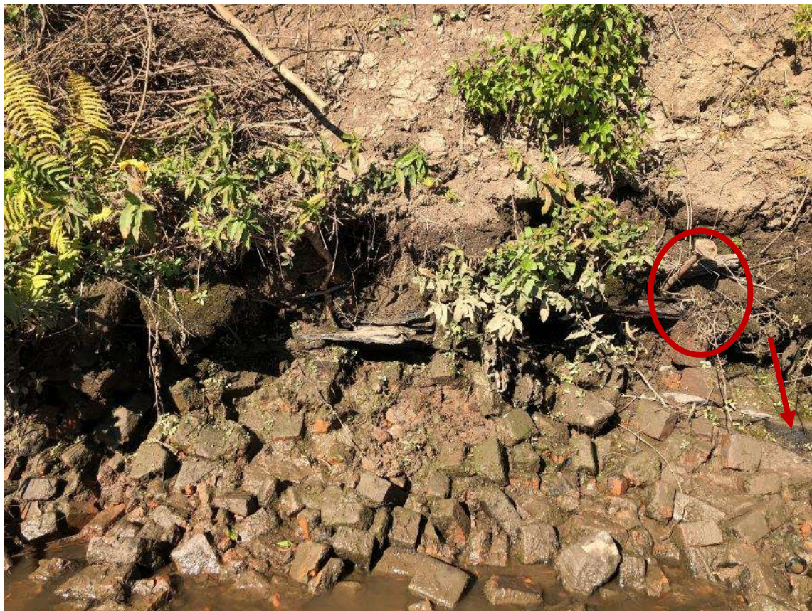
Figure 123: Section of AWF2, showing timber beam with bolt B11 (red circle) and brick rubble pile (AWF13). A cut off pile (AWF2/4) associated with this feature is lower right of frame (red arrow).
