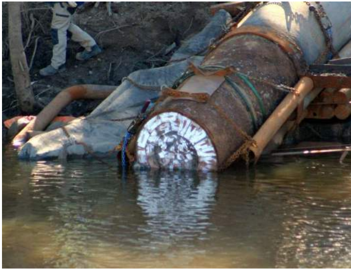
Figure 162: Iron pier removed from 1874 Windsor Bridge during demolition, showing internal brickwork (photograph by Neil Dand, April 2020). 267
