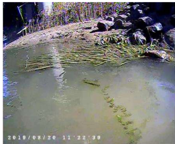
Figure 310: Upstream extent of north side rock armour. (Video: WBRP Rock Armour run 004, still image taken at 06:30)
