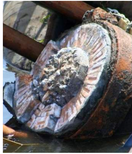
Figure 163: Detail of 1874 Windsor Bridge pier internal brickwork (photograph by Neil Dand, April 2020). 268
