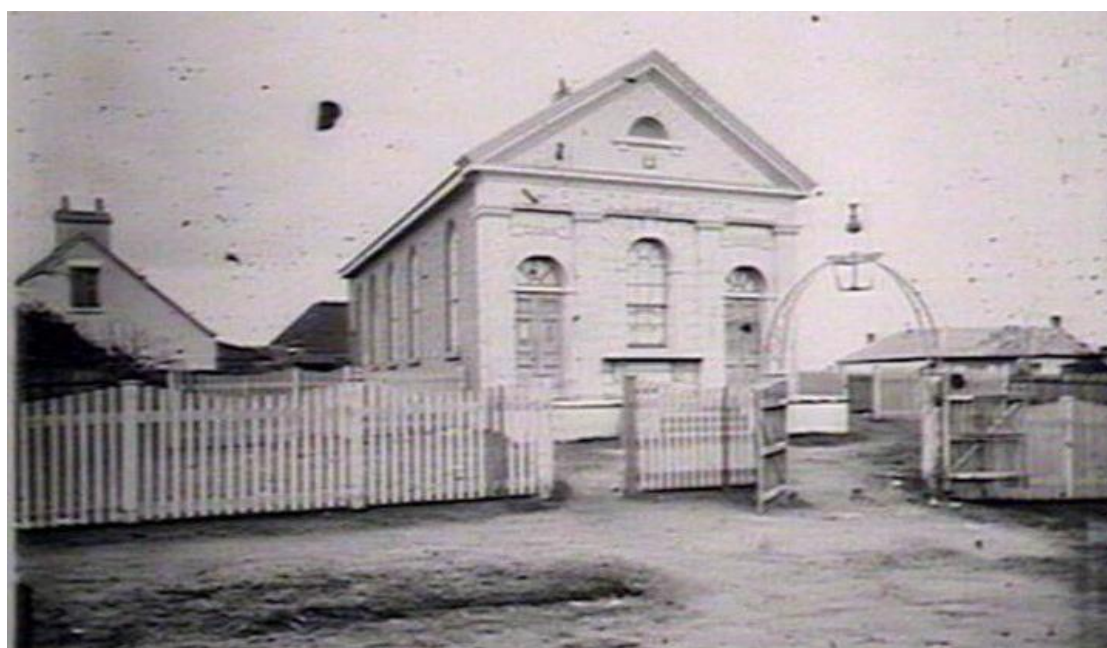
Plate 33: View of the School of Arts in c. 1870 showing the wider property boundary; test trench 10 would lie on the other side of the picket fence within the boundaries of the School (source ML GPO 1-06260.).
