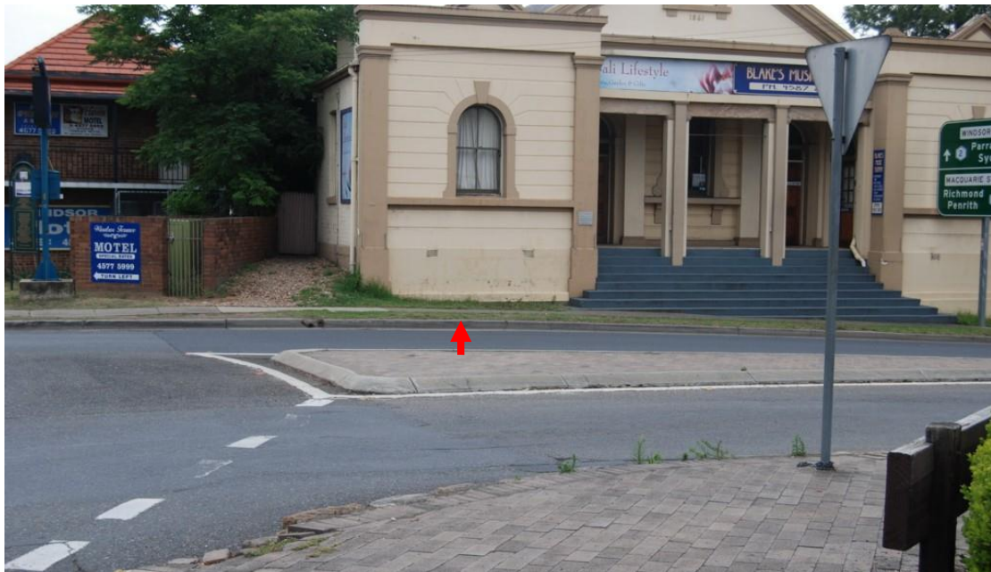
Plate 4: View east showing Bridge Street and the School of Arts building; the position of the test trench is indicated by the arrow
