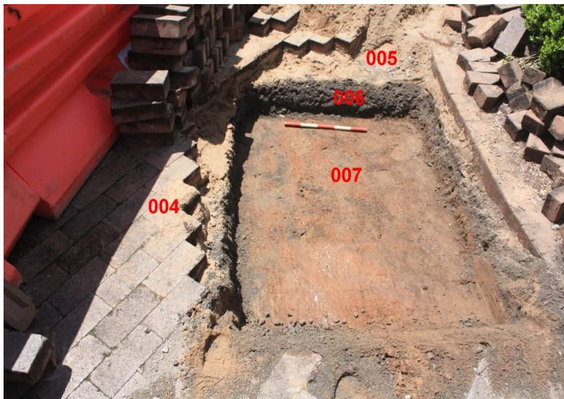
Plate 12: View east of Trench 11 showing the surface pavers and bedding sand and the George Street road surface [006] in section. The base of the trench is covered with a silty soil deposit [007]; scale 500mm
