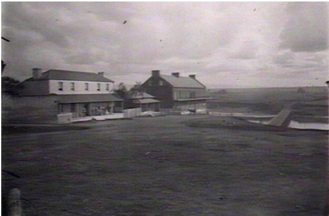
Plate 30: View of the southern end of Thompson Square after 1874 showing the Macquarie Arms Inn and the area of George Street in the foreground (source ML d1-06257)
