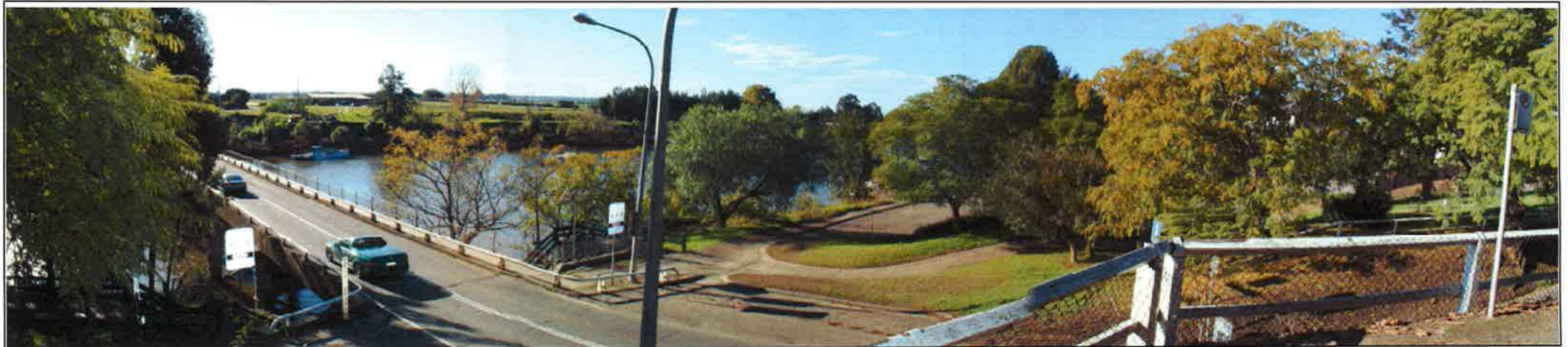
Figure 8: View of the existing Windsor Bridge from Doctor's House, Windsor (Source: RMS 2012)
