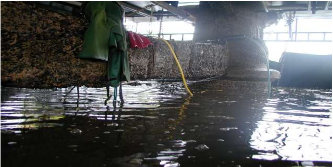
One of the existing lower pier tie beams after removal of reinforcement concrete cover. Note the sheered main reinforcement and stirrups.
