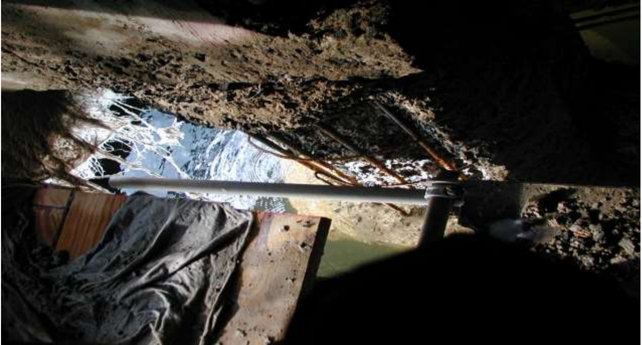
Removal of dilapidated concrete from bridge pier prior to treatment
