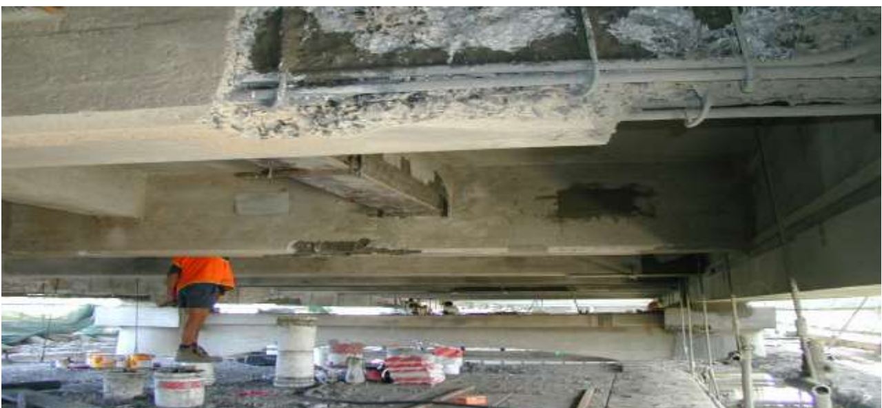
Conventional repair work to the underside of the bridge. Sediment sheets were suspended below to trap loose debris which was then dumped into a barge.
