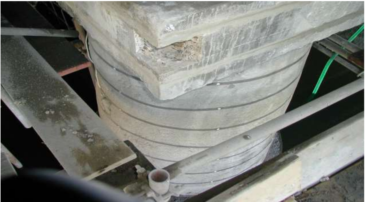
Pier showing application of anode strips as part of the Cathodic Protection work prior to application of final concrete coating.
