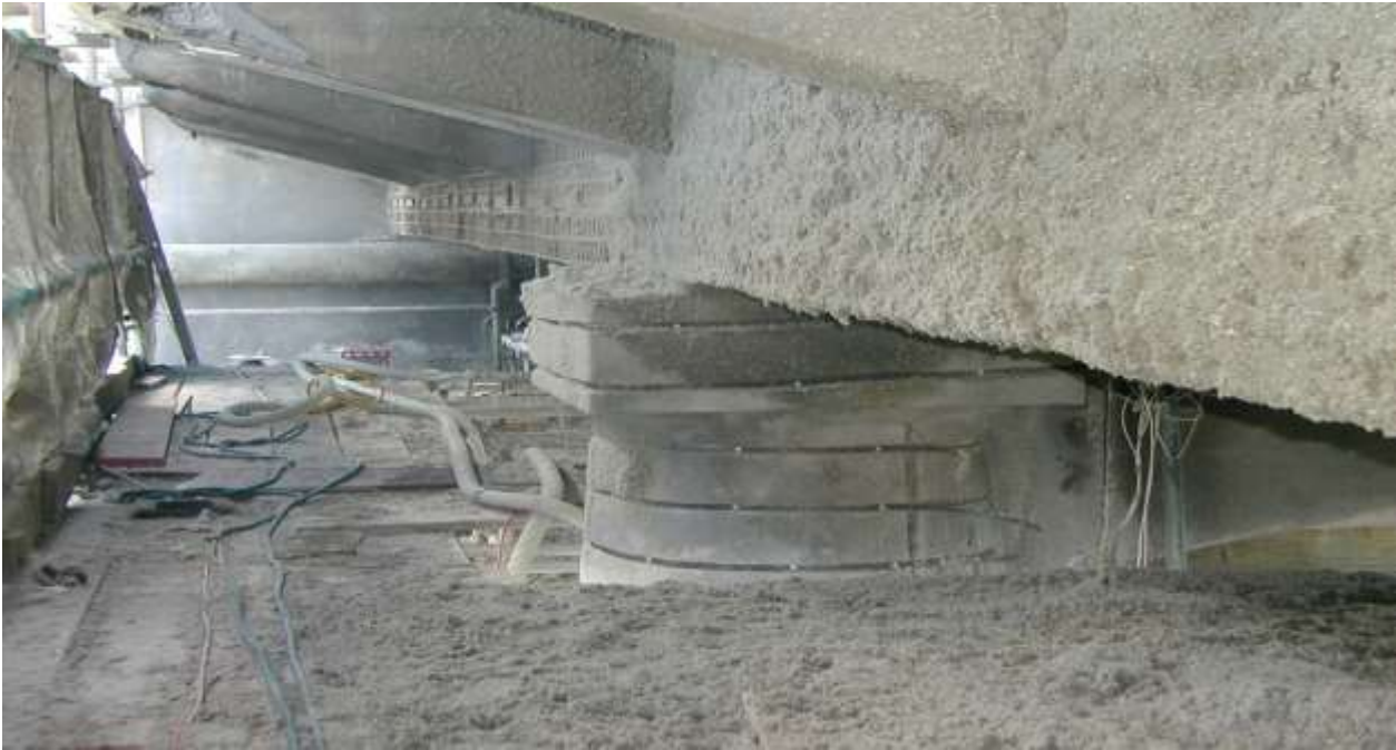
Realkalisation treatment to existing edge beams
