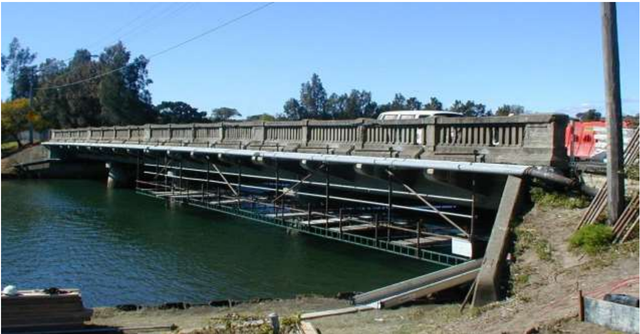
View of the existing bridge structure prior to remedial treatment
