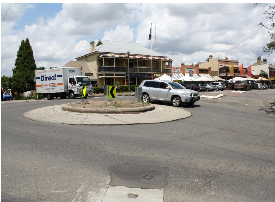
Figure 3-4 George Street / Bridge Street intersection (looking south west)
