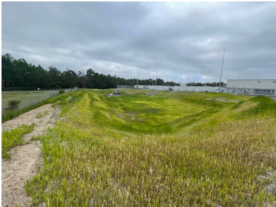
Stabilised sediment dam with outlet structure
