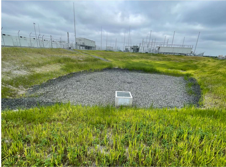
Stabilising sediment dam and outlet structure.
