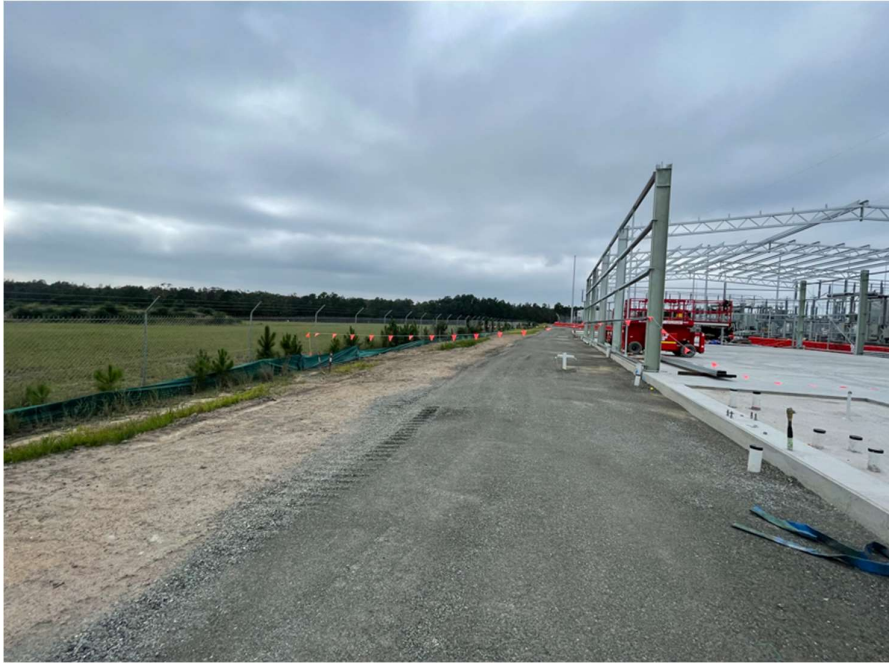
Operations and Maintenance building under construction (right), boundary sediment fence (left)
