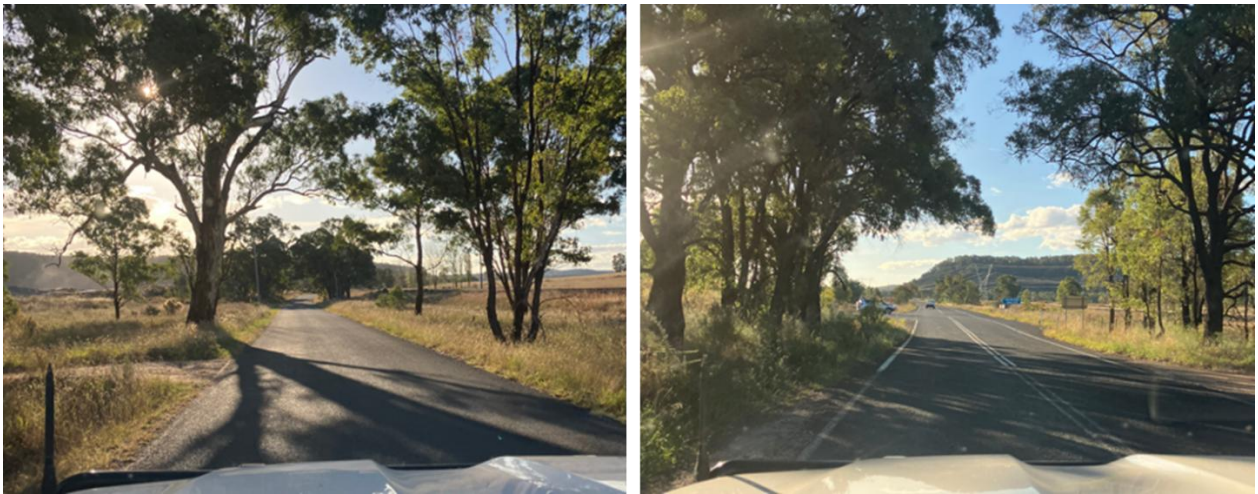
FIGURE 2 ULAN-WOLLAR ROAD (SITE PHOTOS DATED APRIL 2025)
