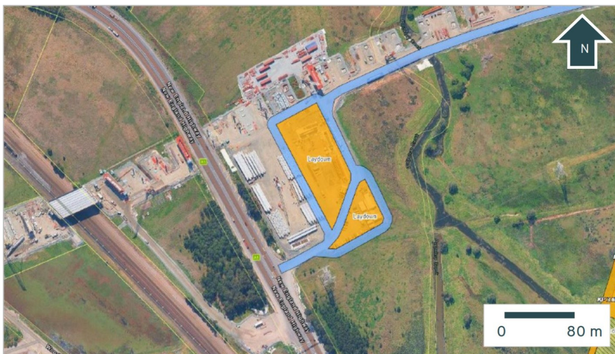
Figure 3.3 Construction laydown and stockpiling area (10/-/DP1150648)
