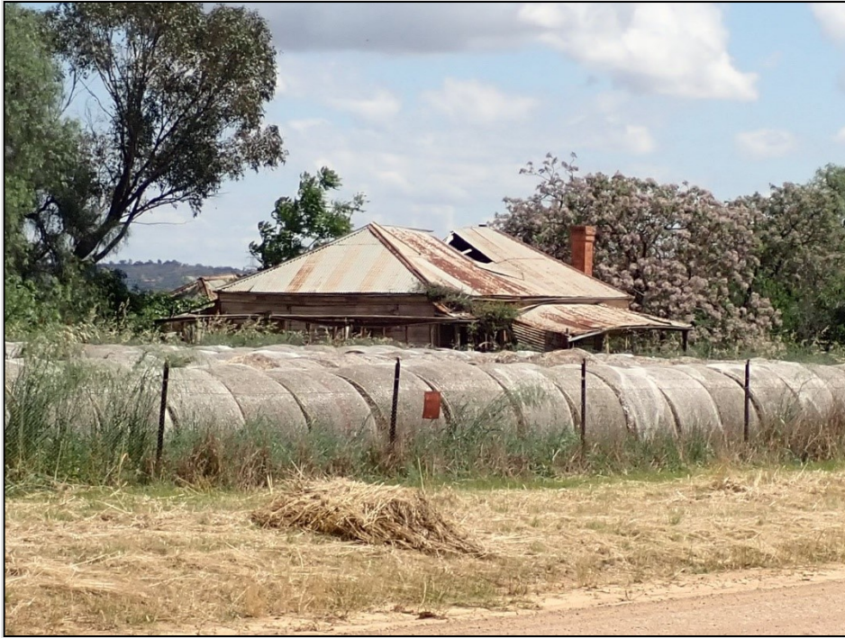
Figure 6-2 View to the Ivydale, north-east from Ivydale Road
