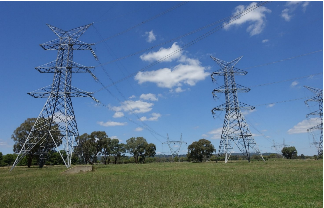
Figure 3-4 Example of 330 kV transmission line structures
