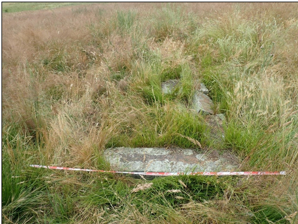
Figure 6-18 Sheep Dip structure, view east
