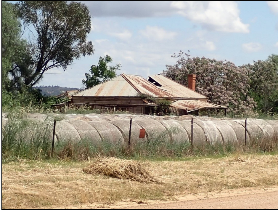
Figure 6-2 View to the homestead, north-east from Ivydale Road
