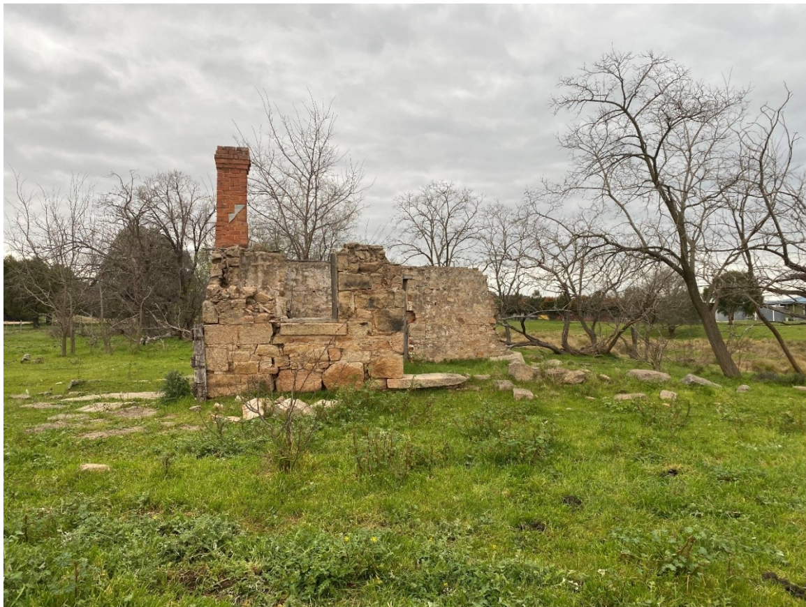
Figure 6-5 Stone Ruin, looking west from Gregadoo Road
