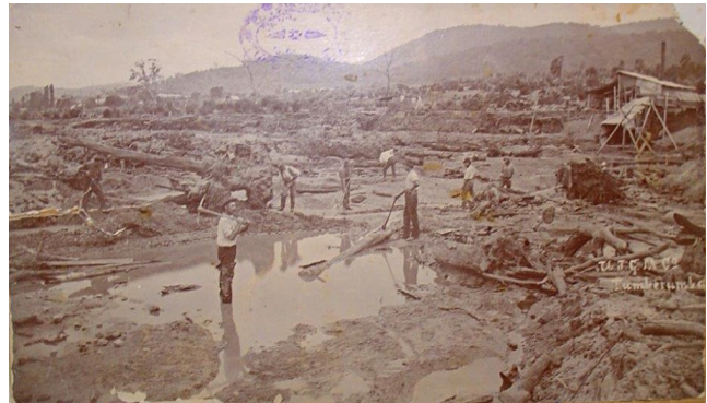
Figure 5-29 Sluicing operations of the Union Jack Gold Mining Company at Tumbarumba Creek, demonstrating the extent of environmental destruction along a creek line 192
